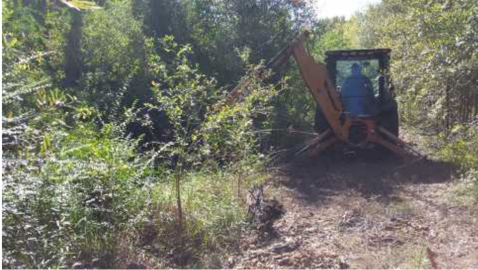
Photo #5: Southerly view of BHT 2 at the onset of excavation.
