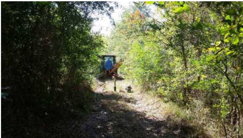
Photo #6: Southerly view of BHT 2 excavation.
