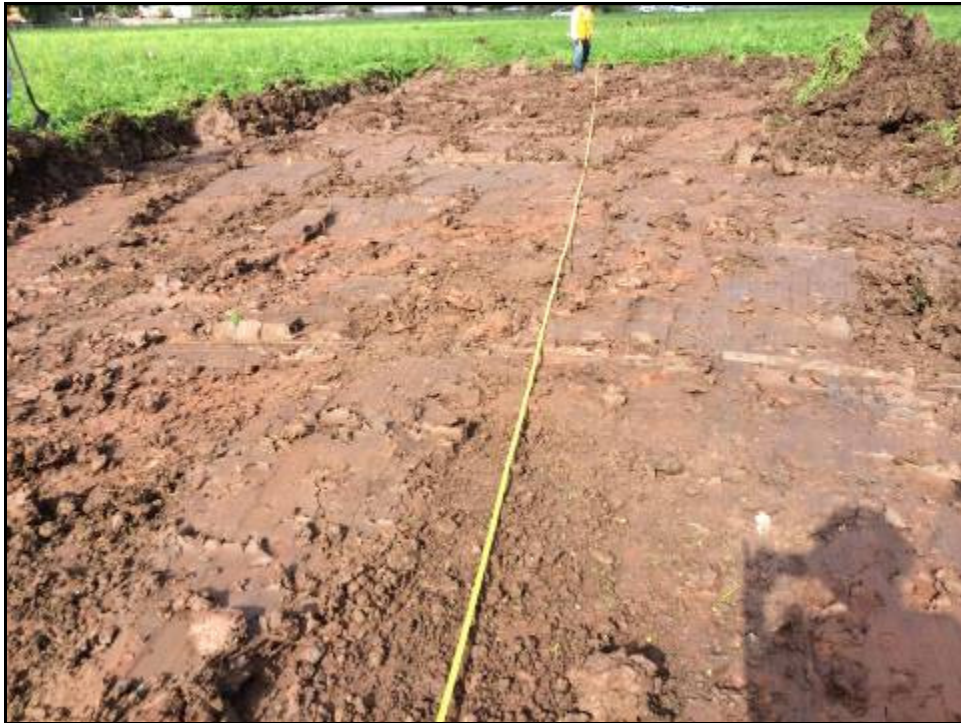
Figure 33: Third 7m-8m x 21m Mechanical Scrap Area
