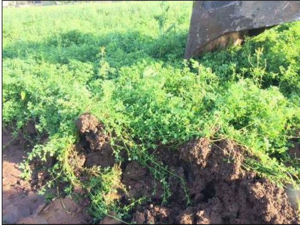
Figure 30: Shallow Trench Showing Disturbed and Intact Soil
