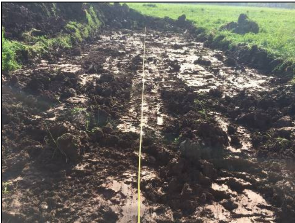
Figure 31: First 7m-8m x 21m Mechanical Scrap Area
