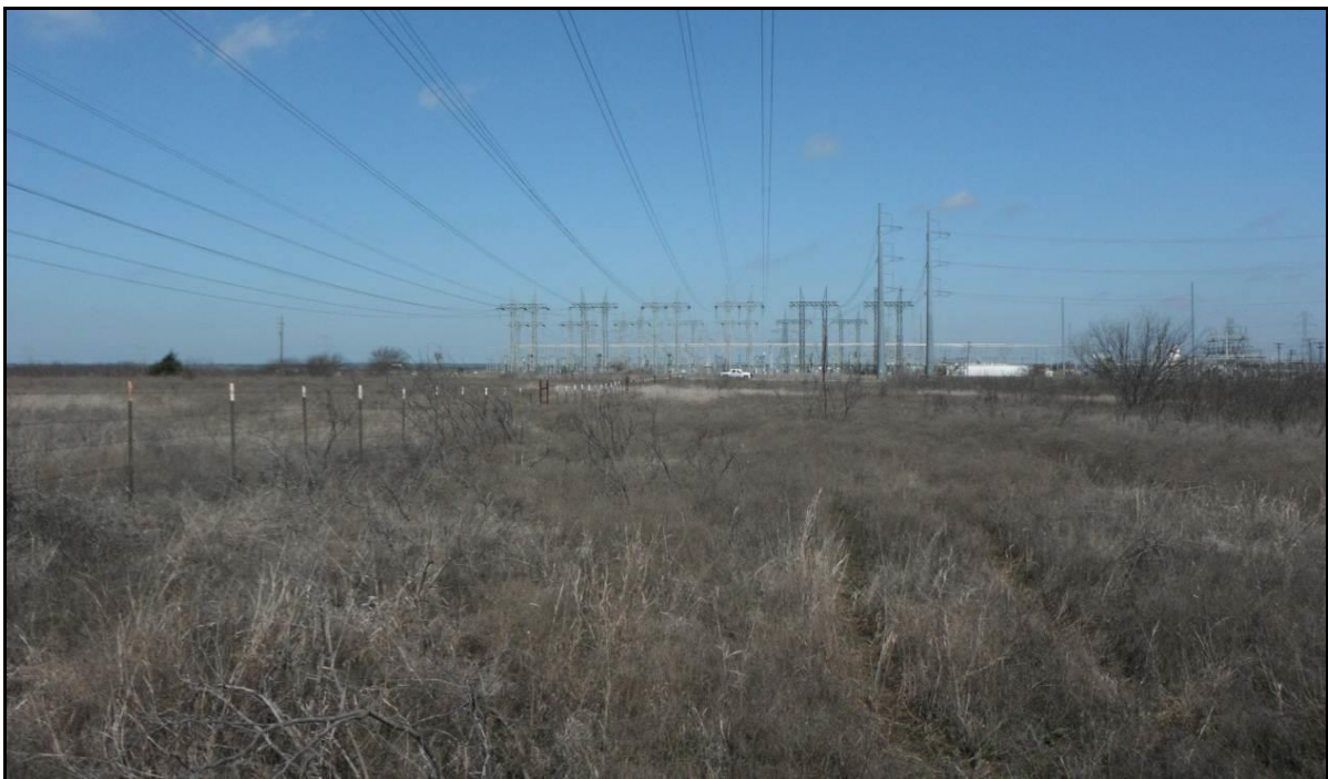
Figure 2-4. View of the transmission lines bordering the Project Area, facing northwest
