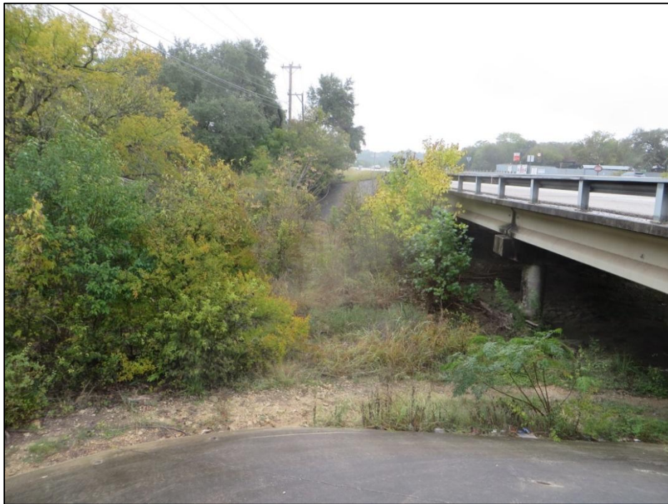
Figure 2-3. Concrete aprons protecting bridge footings on both sides of Helotes Creek
