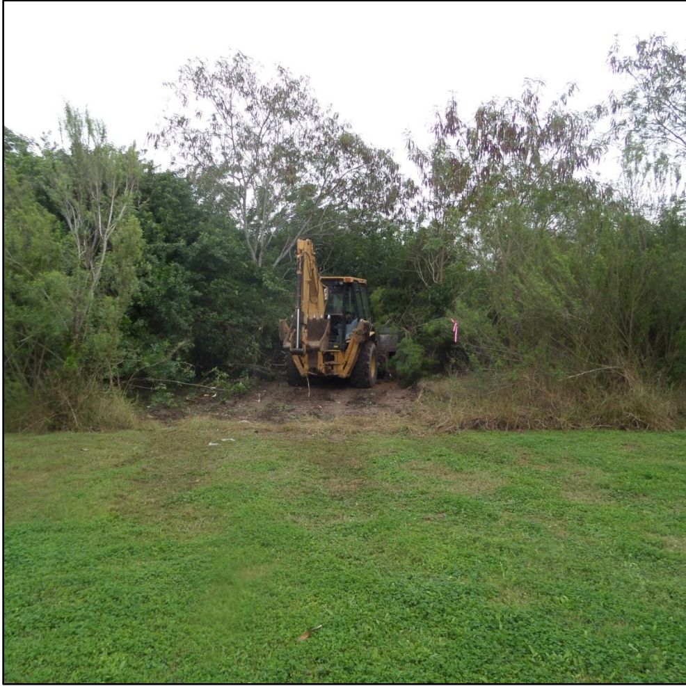
Figure 5-3. Area of vegetation removed in order to excavate BHT 1.
