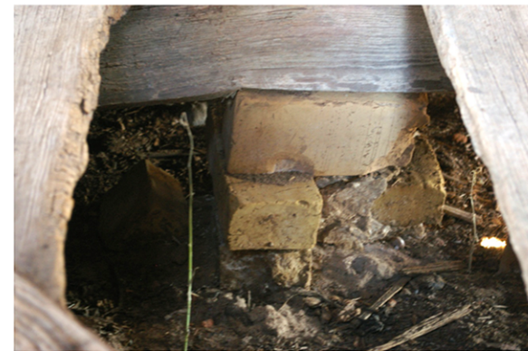
g) Detail of handmade bricks likely supporting former wood burning stove.
