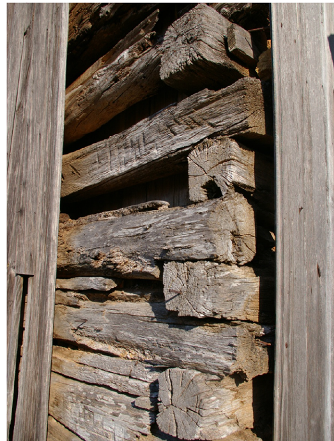
f) Corner notching detail of log house core.
