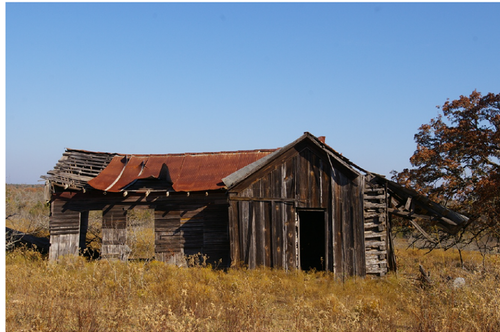
a) View of north elevation, camera facing south.
