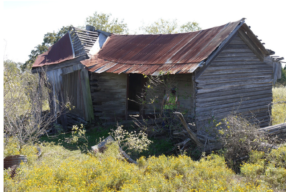
b) View of northwest oblique, camera facing southwest.
