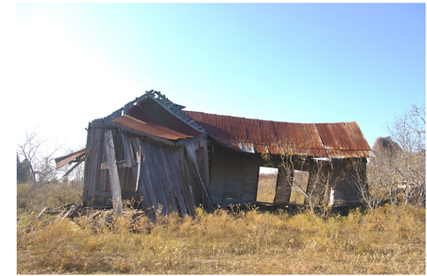
c) View of south elevation, camera facing north.
