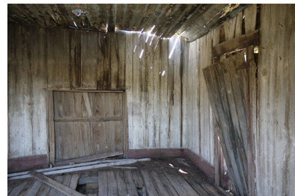
h) Log house interior. Note closed chimney gap and hole in ceiling for wood burning stove.
