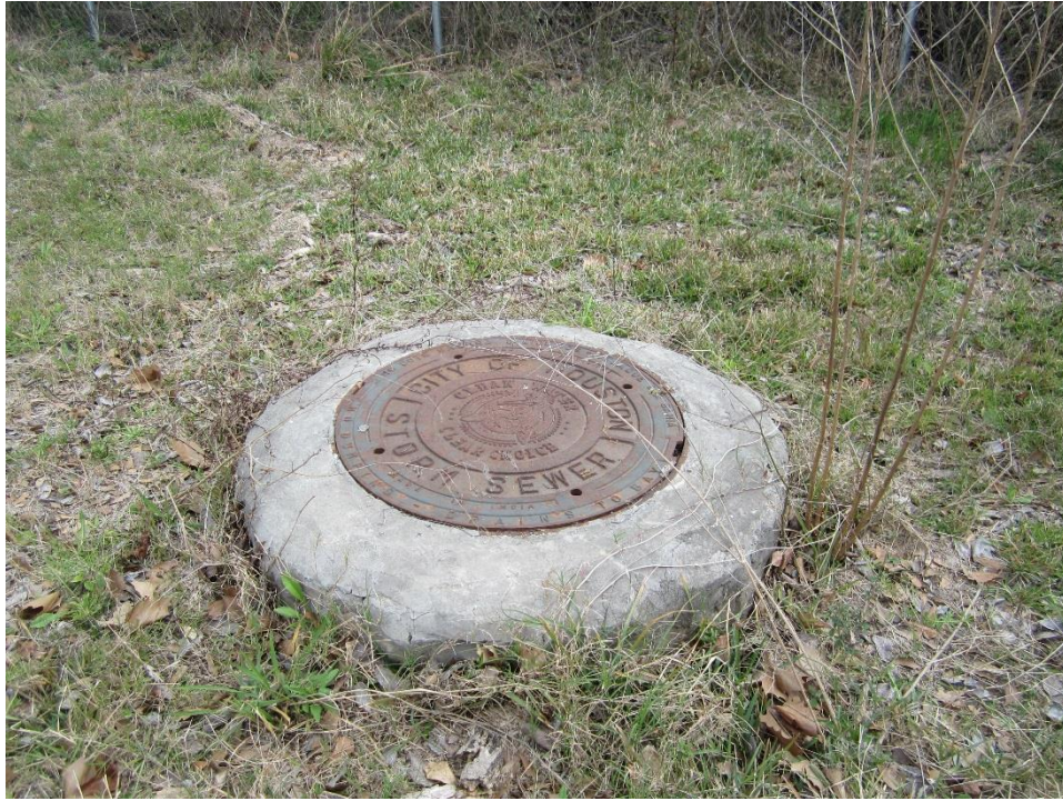
Figure 5-6. Sewer manhole at right angle turn of proposed hike and bike trail corridor on Mercer Arboretum property.
