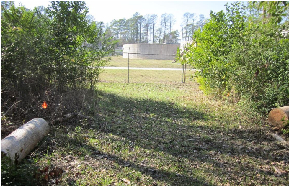
Figure 5-2. View of the Timber Lane Wastewater Treatment Plant, looking west.
