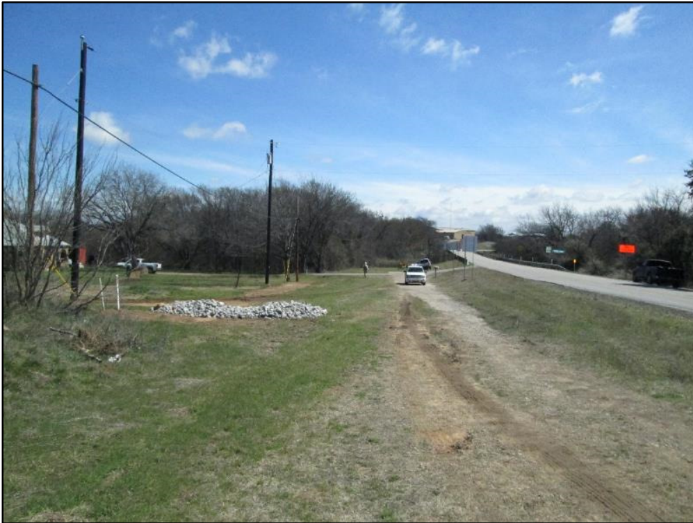
Figure 7. Northwest quad of bridge replacement, facing east toward Hog Creek.
