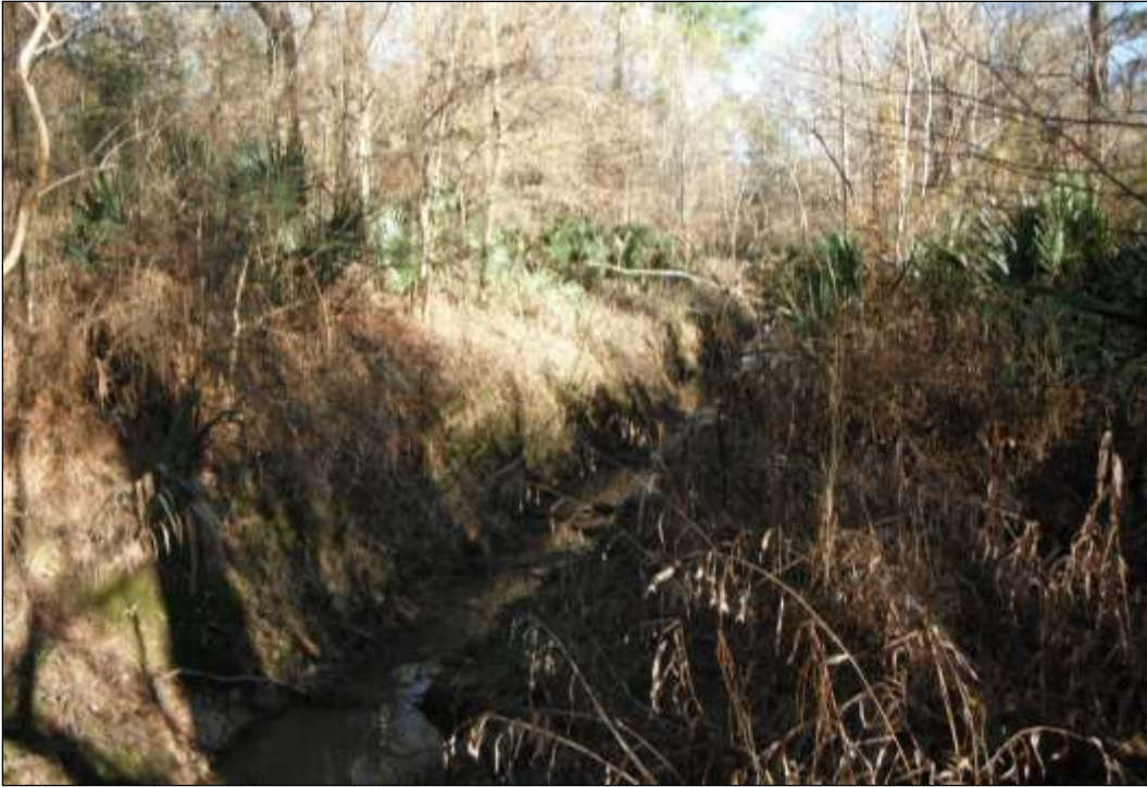
Figure 4. Typical View of Artificial Diversion Canal (Facing Southwest)
