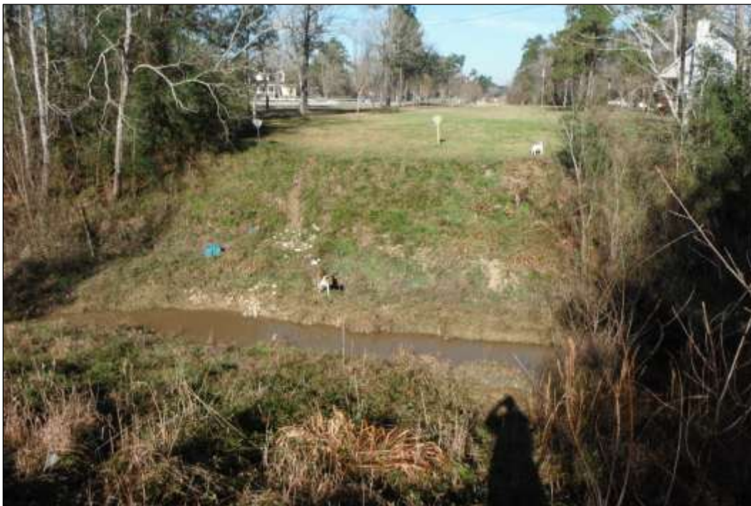
Figure 7. Contoured Portion of Coon Marsh Gully at Pipeline Crossing (Facing Northwest)
