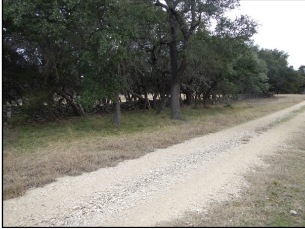
Figure 10. Overview photo of rock wall, facing west/southwest.
