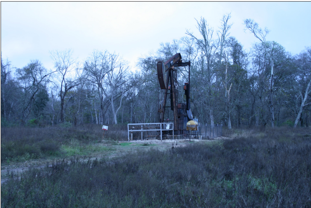
Photo 4. An active oil pumpjack west of the oil field road, whose infrastructure disturbs the survey corridor; view to the north.
