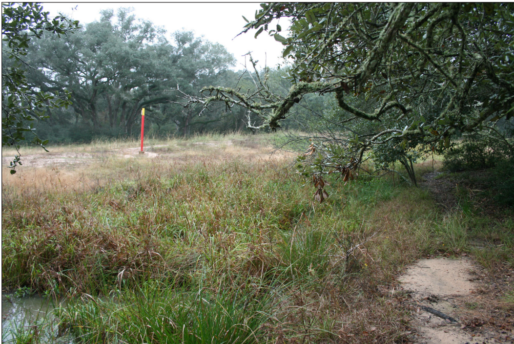
Photo 2. Heavily modified canal and levee, view to the south-southwest.
