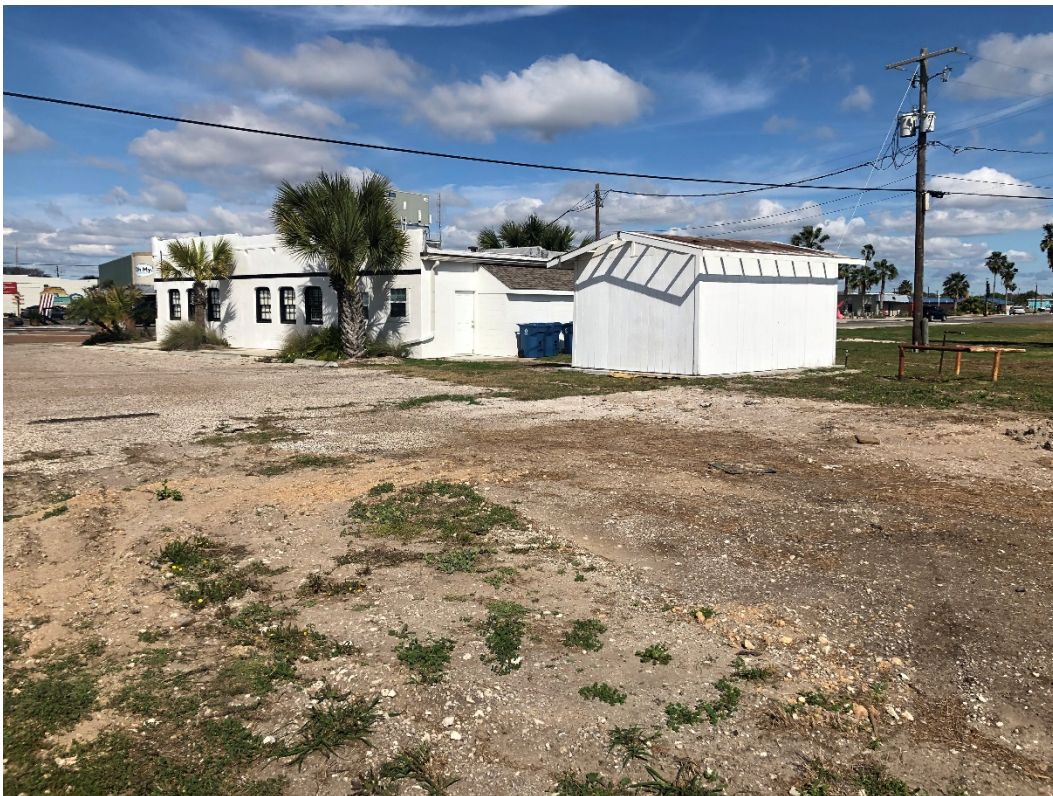
FIGURE 11. VIEW OF NORTHERN HALF OF APE, FACING NORTHWEST
