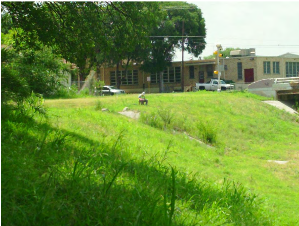
Figure 22: Overview of Project Area facing west from STJH5 towards archeologist at STDK4.
