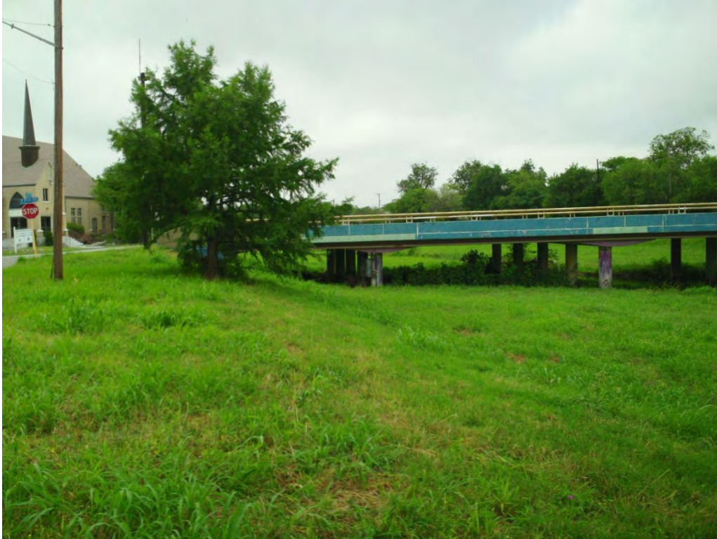
Figure 16: Overview of Project Area facing west towards Woodlawn Street Bridge.
