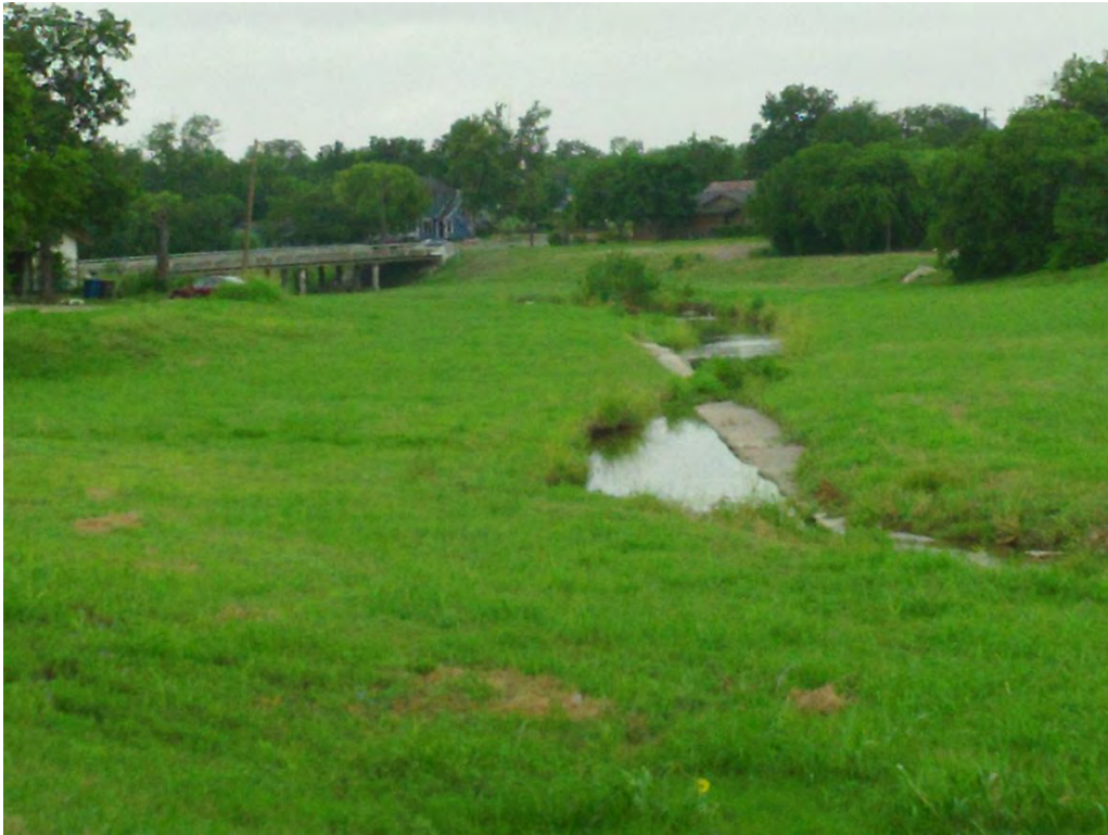
Figure 17: Overview of Project Area facing west towards Cincinnati Street Bridge from STJH4.
