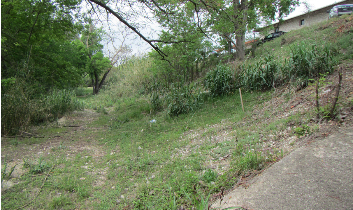
Figure 2. View to the west of the Jefferson Street force main corridor from the Water Street bridge. Town Creek and the existing sewer line access road are to the left, and a parking lot atop introduce fill is to the right.
