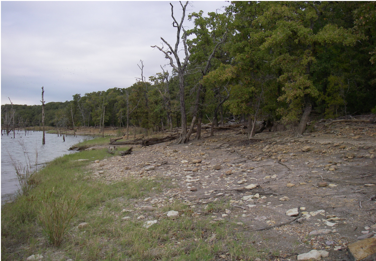
Figure 12. View of erosion within 41HI150–153, typical of most sites along the lake margins.
