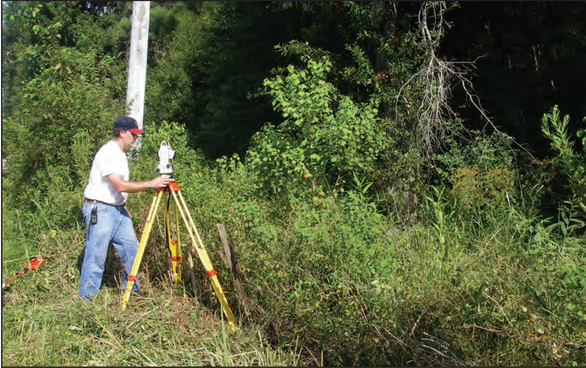
Figure 6-2. Setting up the Sokkia total station at the edge of the barbed-wire fence that runs along the northern edge of the current IH-10 ROW adjacent to the north tract. A line was cut from this location to the north, through the dense woods to the right, for a distance of 28.10 m to the southeastern corner of the area to be cleared.
