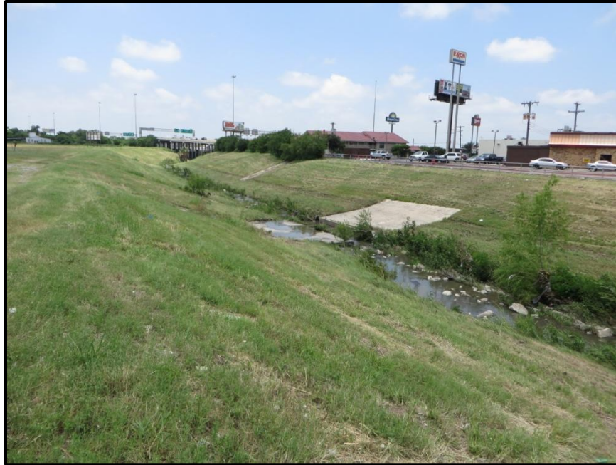
Figure 1-3. Graded San Pedro Creek banks south of FM 536 (South Alamo Street).
