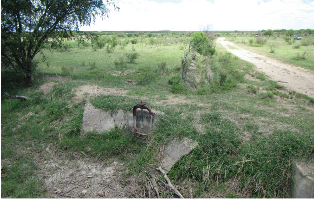
Figure 35. Photograph of headgate that allowed water to enter lateral ditches from the main channel in the Kincaid irrigation system.
