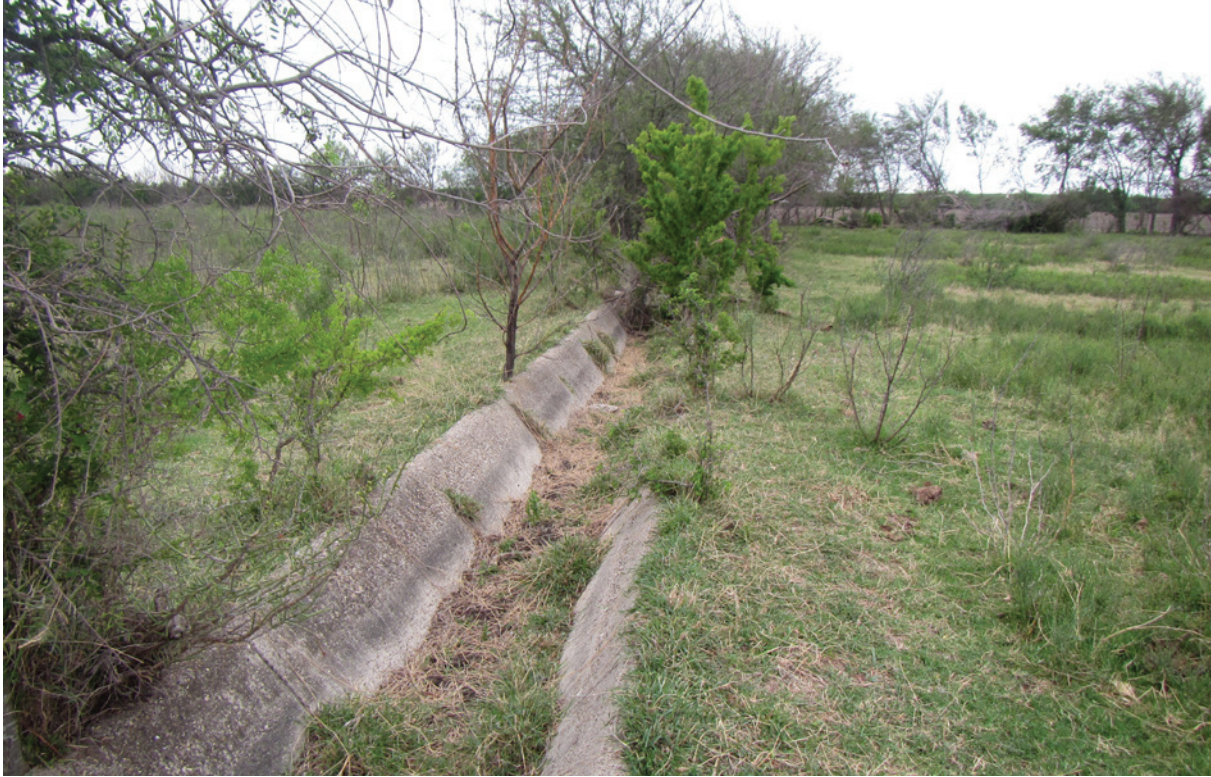
Figure 33. Photograph of ditch along the Kincaid irrigation system overgrown with foliage. This lateral ditch delivered water to manmade terraces on the Elm Creek floodplain.
