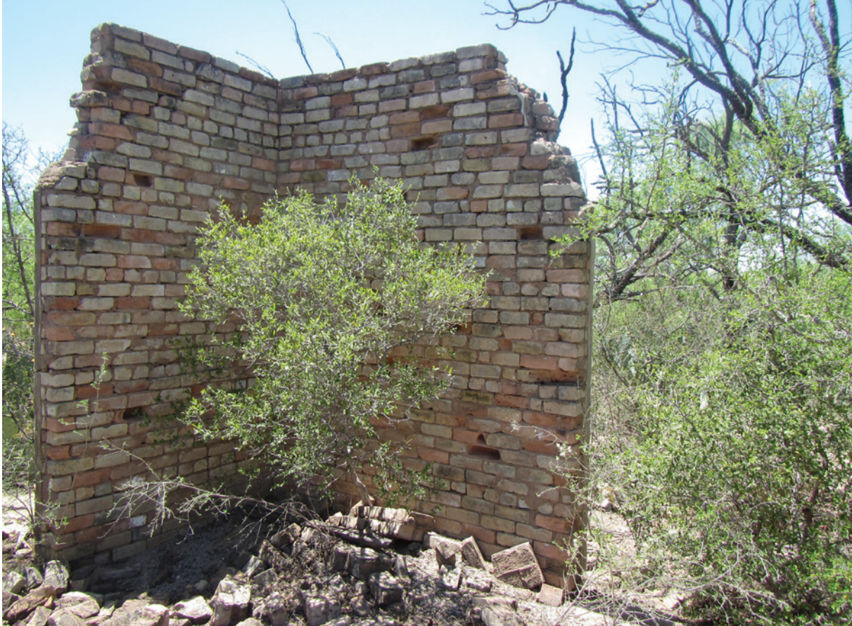
Figure 13. Remnant walls of the ruinous hunting lodge at 41MV389 indicate early-twentieth-century construction with their handmade bricks and soft mortar joints.
