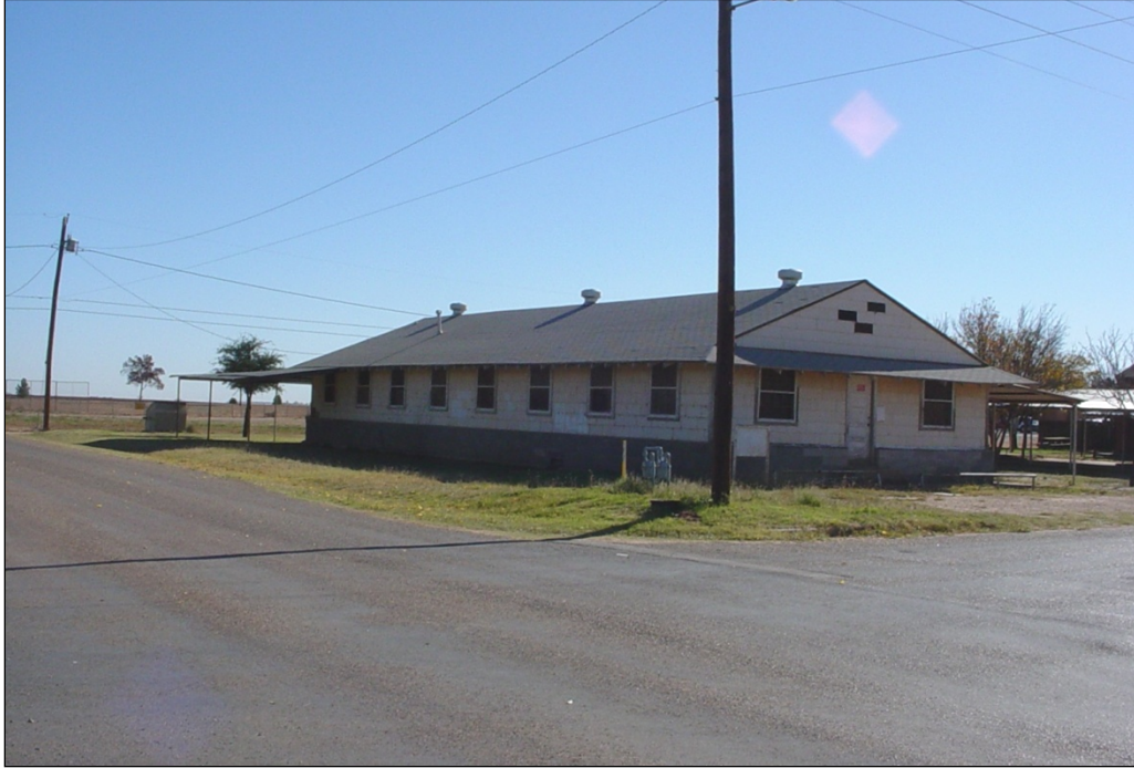
Figure 13. Structure at 4th Street and Hartford Avenue. Iowa Street is visible in the background (frame left).
