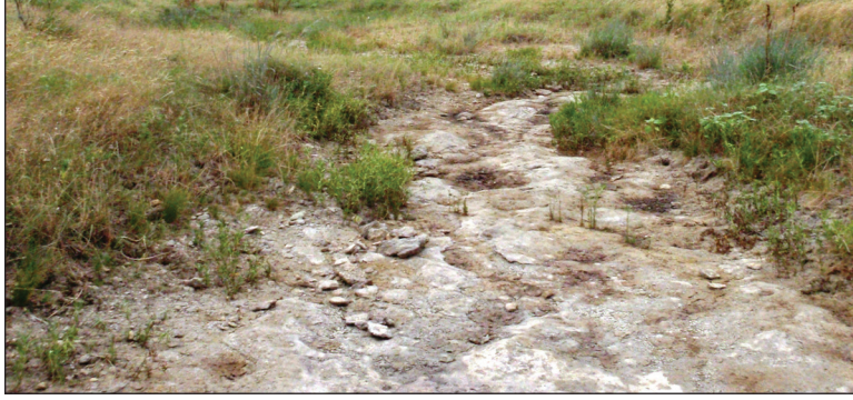
Figure 5. Visible erosion on ground surface.
