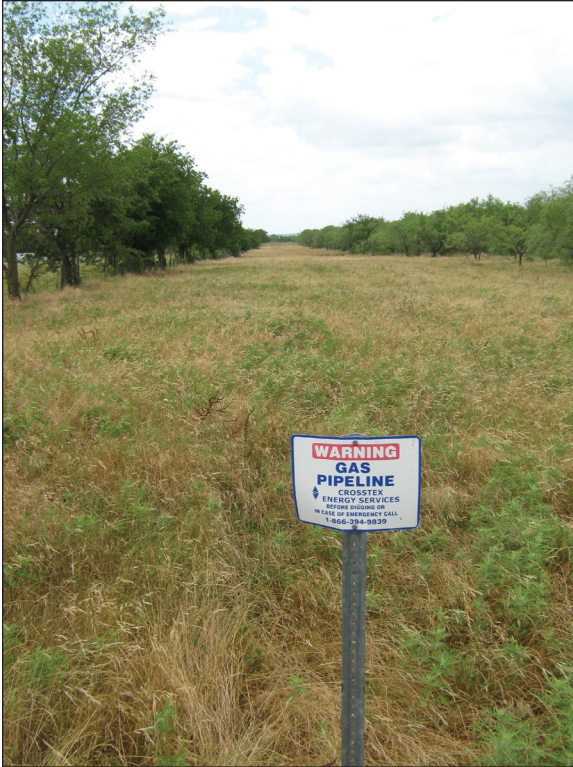
Figure 10. Cleared vegetation overlying the pipeline corridor.
