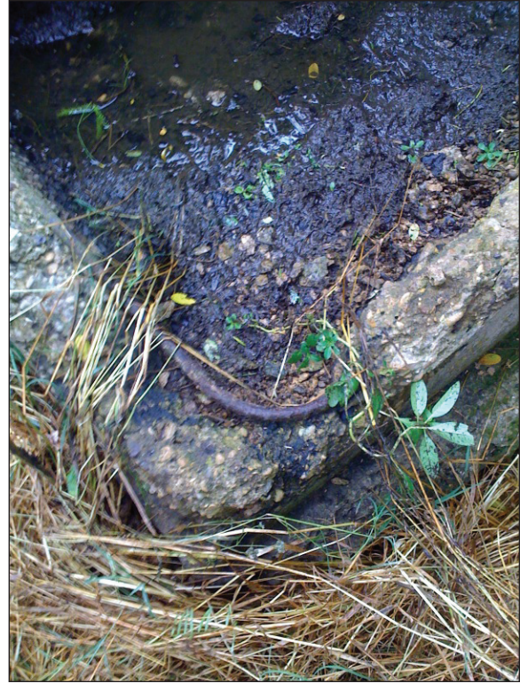
Figure 14. Grooved iron rebar within water trough.
