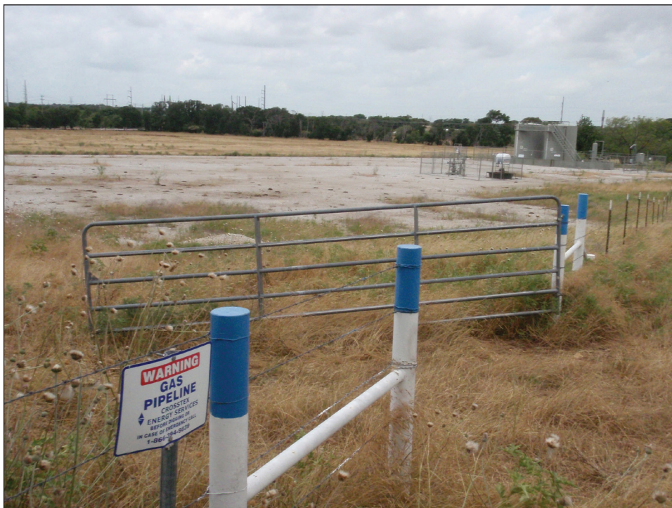
Figure 11. Devon Energy Production facility.
