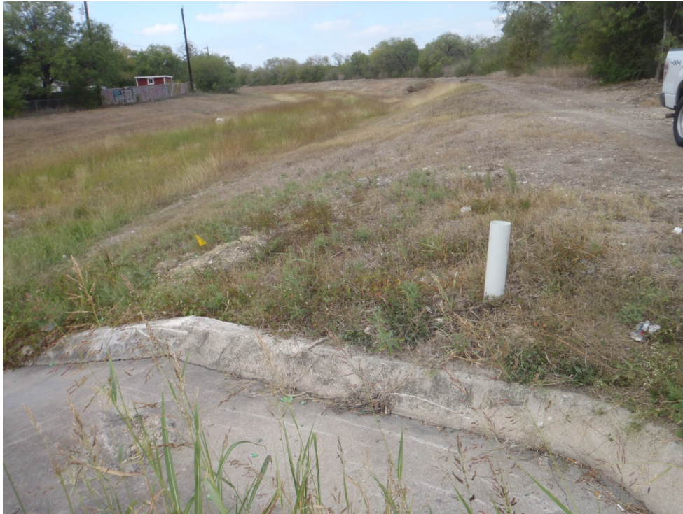
Figure 7. Channelization of Indian Creek within Survey Area 3, facing northwest.
