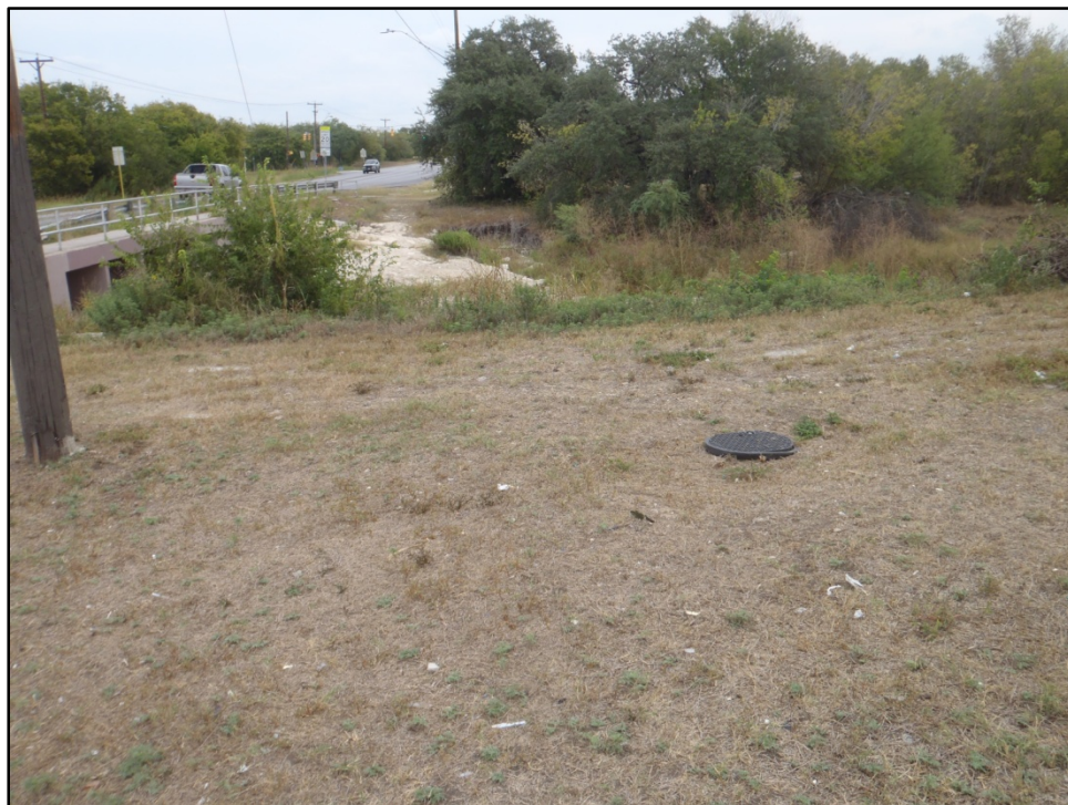
Figure 8. Sanitary sewer and overhead utilities in Survey Area 4, facing northeast.
