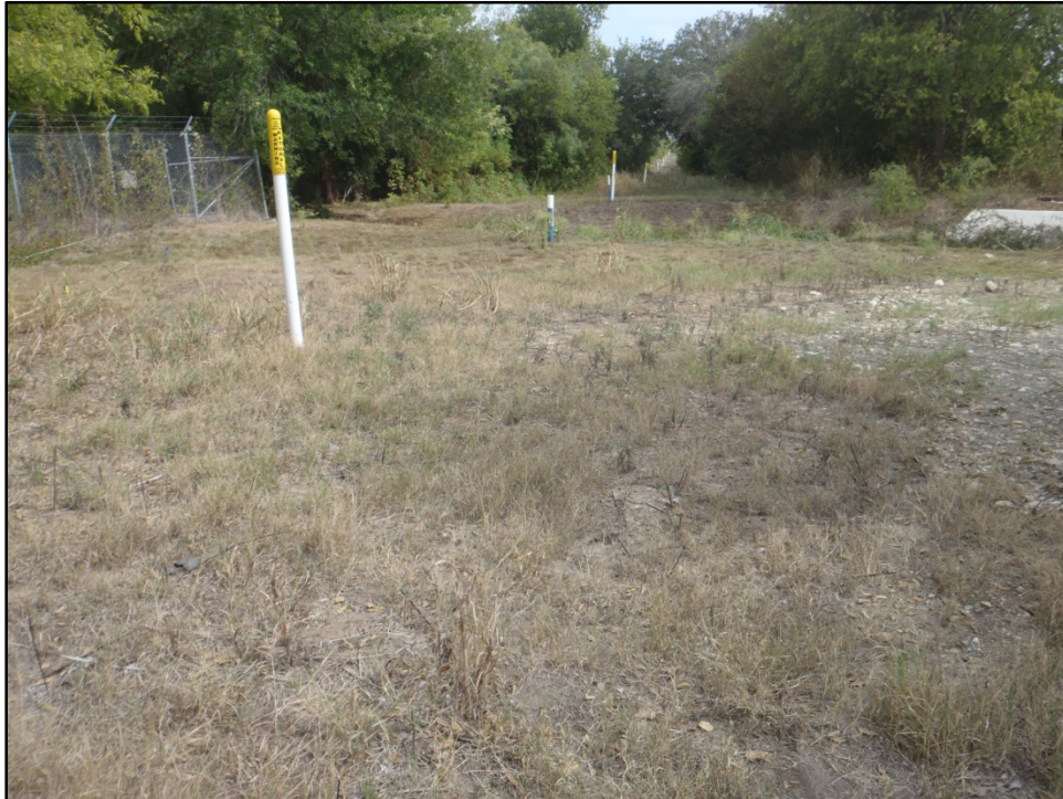
Figure 6. Survey Area 2 consisted mainly of an easement for a high-pressure underground gas pipeline, facing east.
