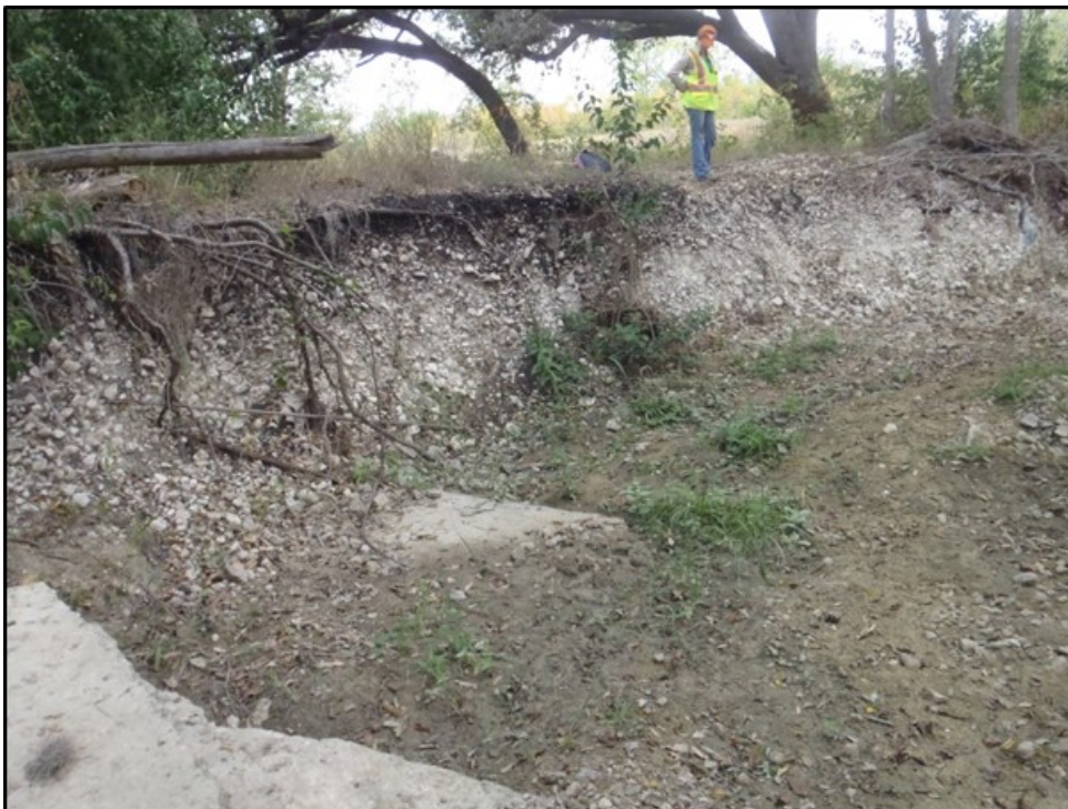
Figure 4. Left bank of Indian Creek within Survey Area 1, facing northeast. Note the erosion and unsorted gravels and cobbles evident in the profile.
