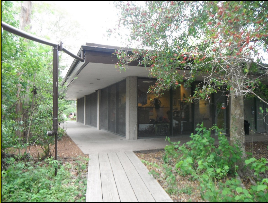
Figure 8. Western square of the Visitor Center, facing northeast.
