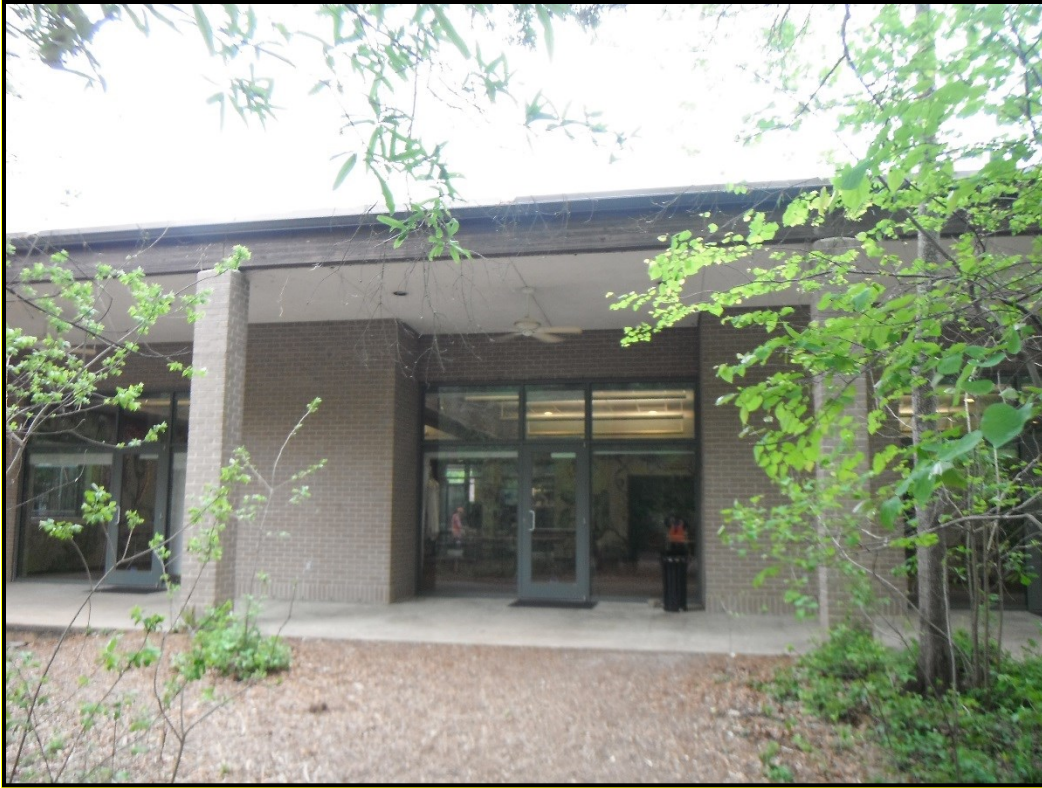
Figure 9. Eastern square of the Visitor Center, facing north.
