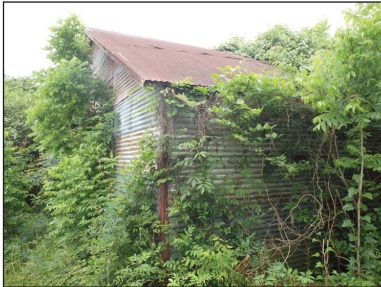
Plate 9. View of Historic-Age Resource #1 within Area C. View is to the west.
