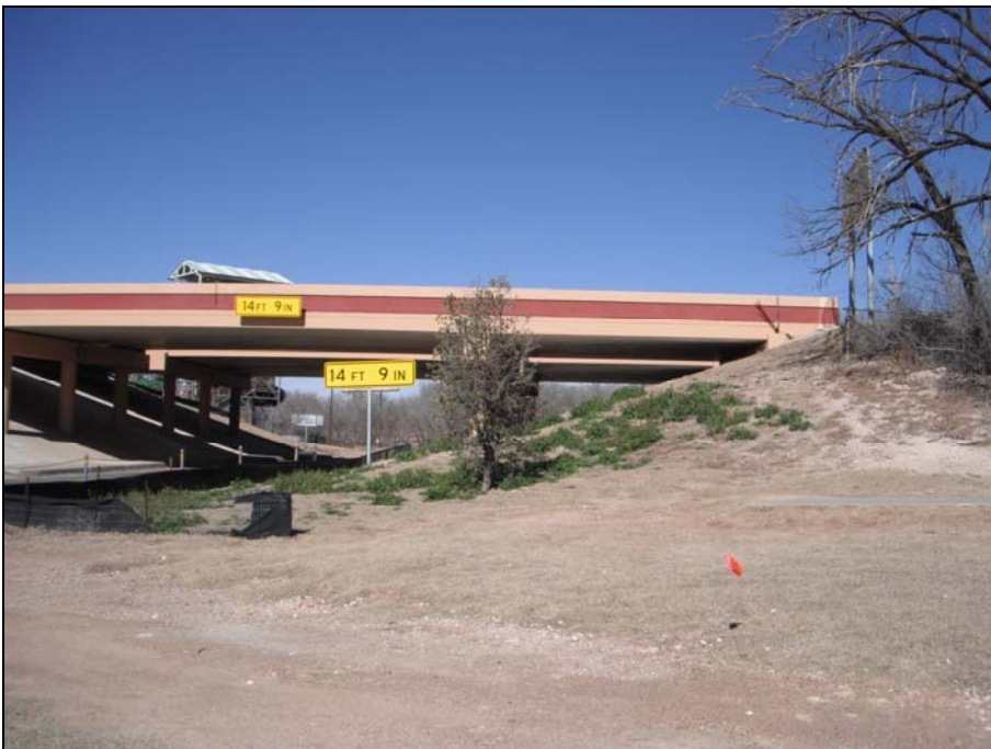
Photo 13. Proposed location of Segments 6 and 7, facing north from south end.
