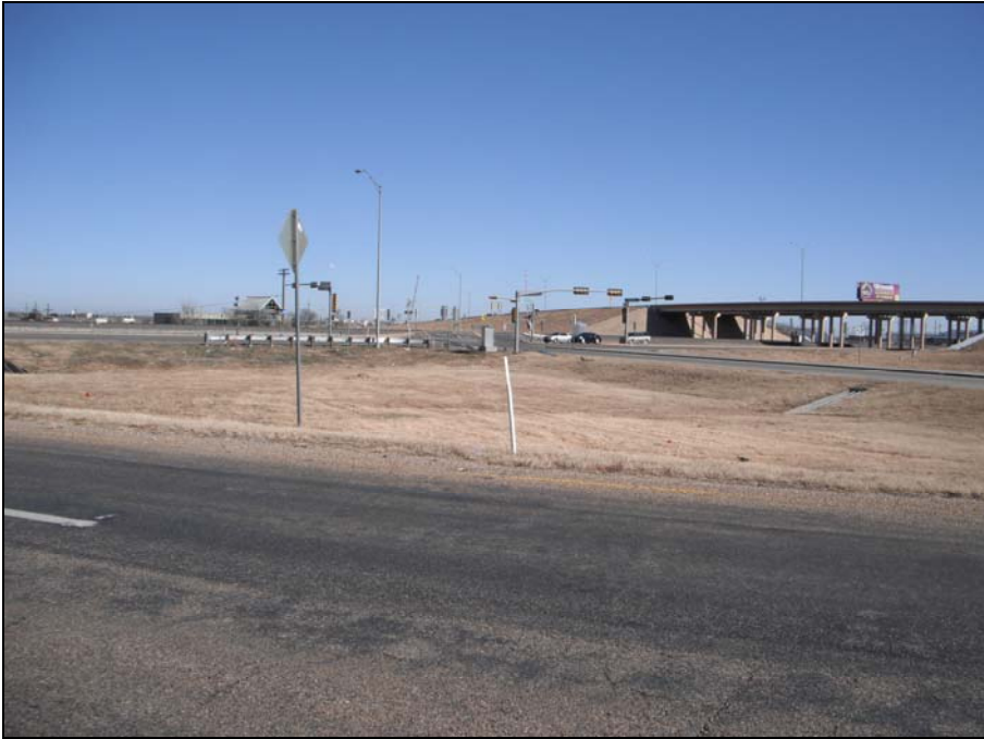
Photo 24. Proposed location for western portion of Segment 18, facing east.
