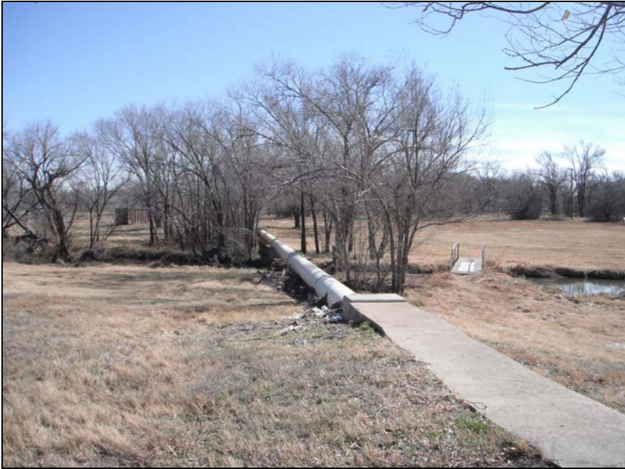
Photo 9. Segment 5, aerial portion, facing south from north side of tributary.
