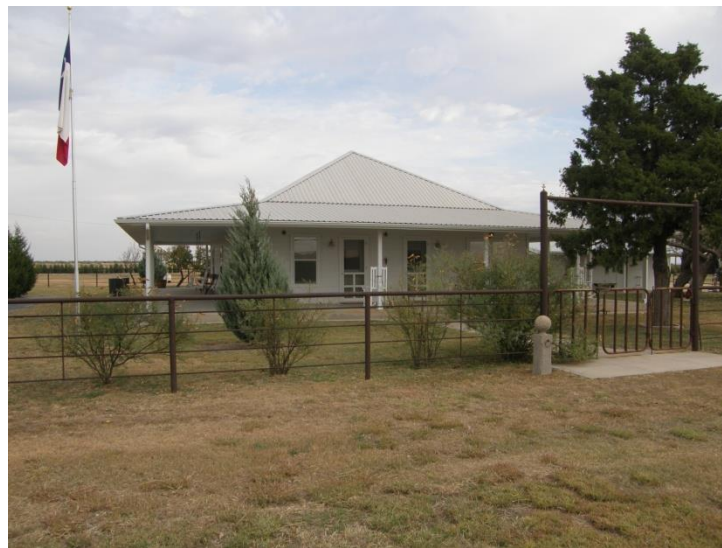
View of the Front of the Ranch House, facing North
