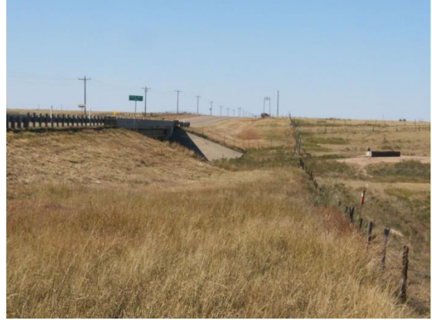
Segment 4 along Hwy 86
