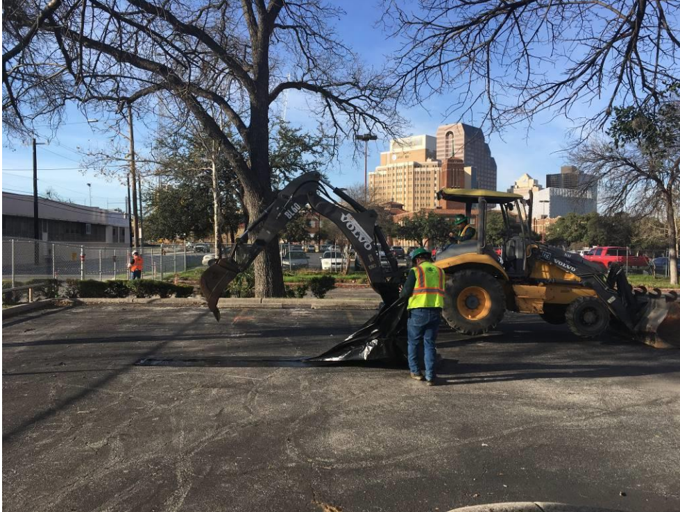
Photo #1: Southwesterly view across the beginning of BHT 1 excavation.
