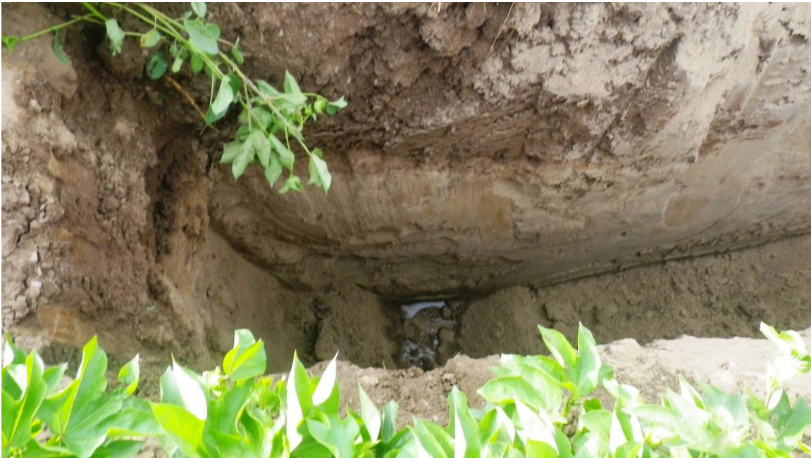
Figure A-9. Water table at the bottom of Trench 1.
