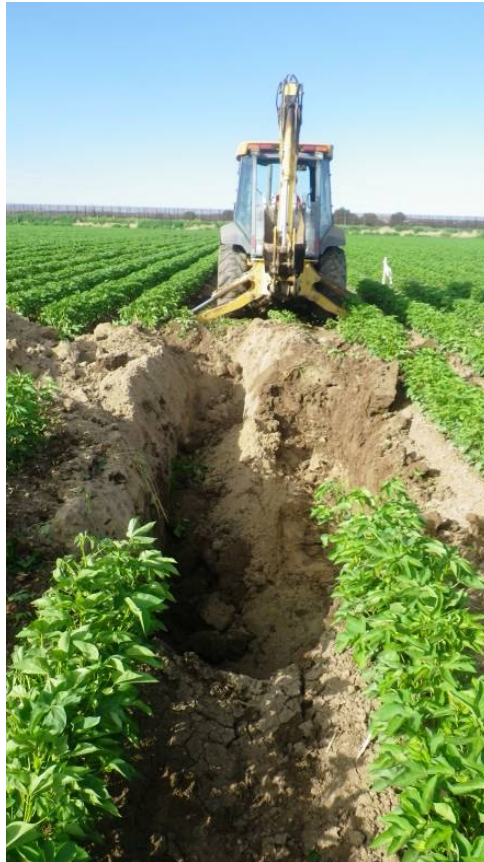
Figure A-10. Overview of Trench 2 looking south.
