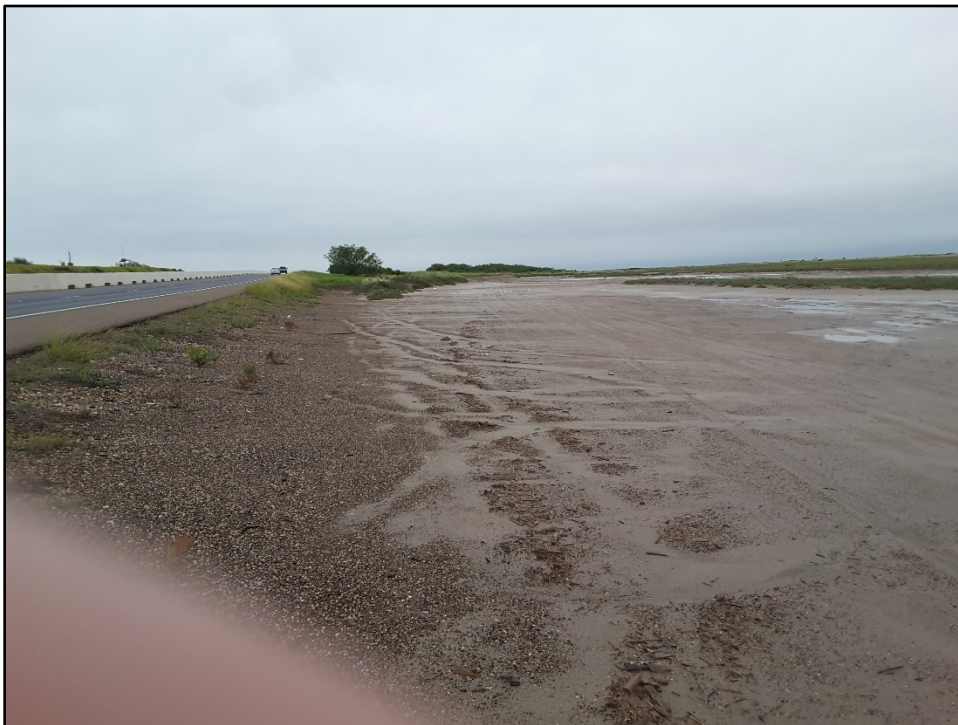
Figure 14. Access road point on tract ND-CAM-082.000 disturbed by previous pipeline construction, facing east.
