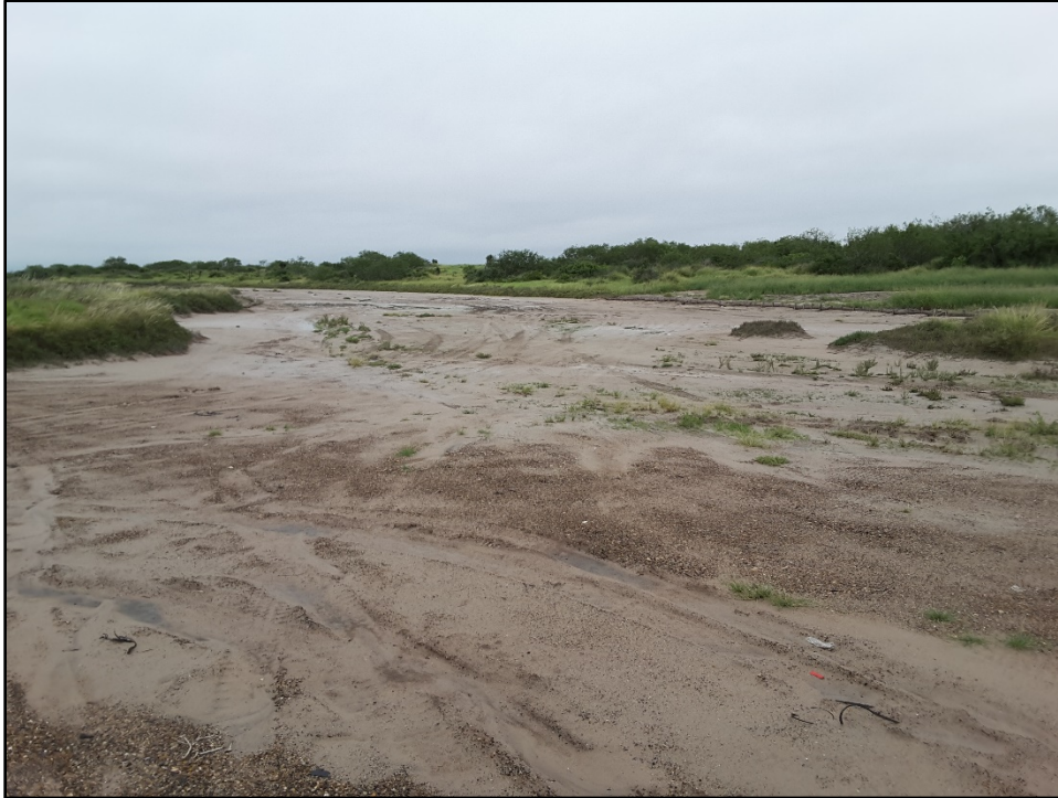
Figure 15. Access road point on tract ND-CAM-082.000 disturbed by previous pipeline construction, facing southeast.
