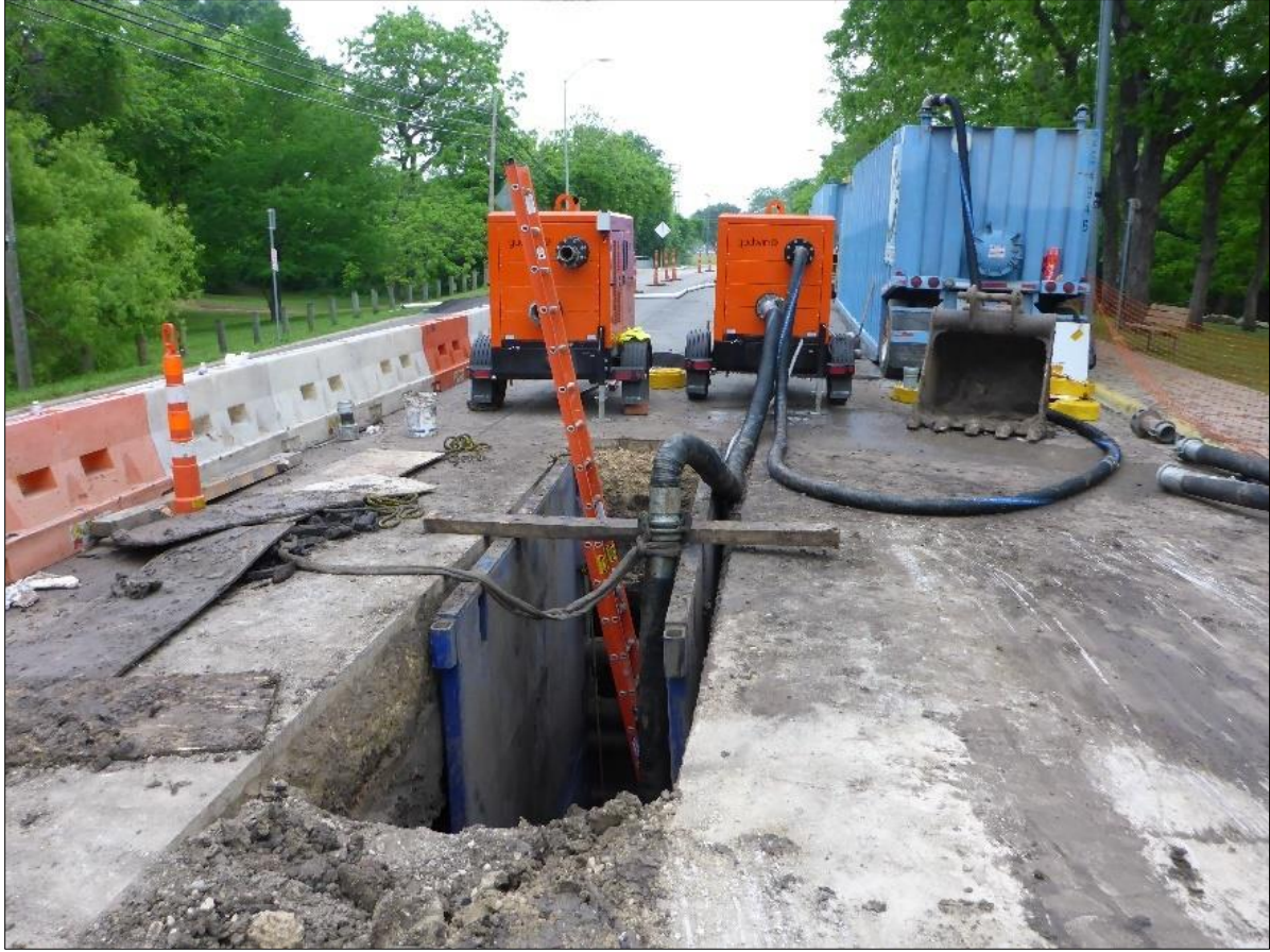
Figure 13. The Drill Rescue Trench, on May 2 nd .
