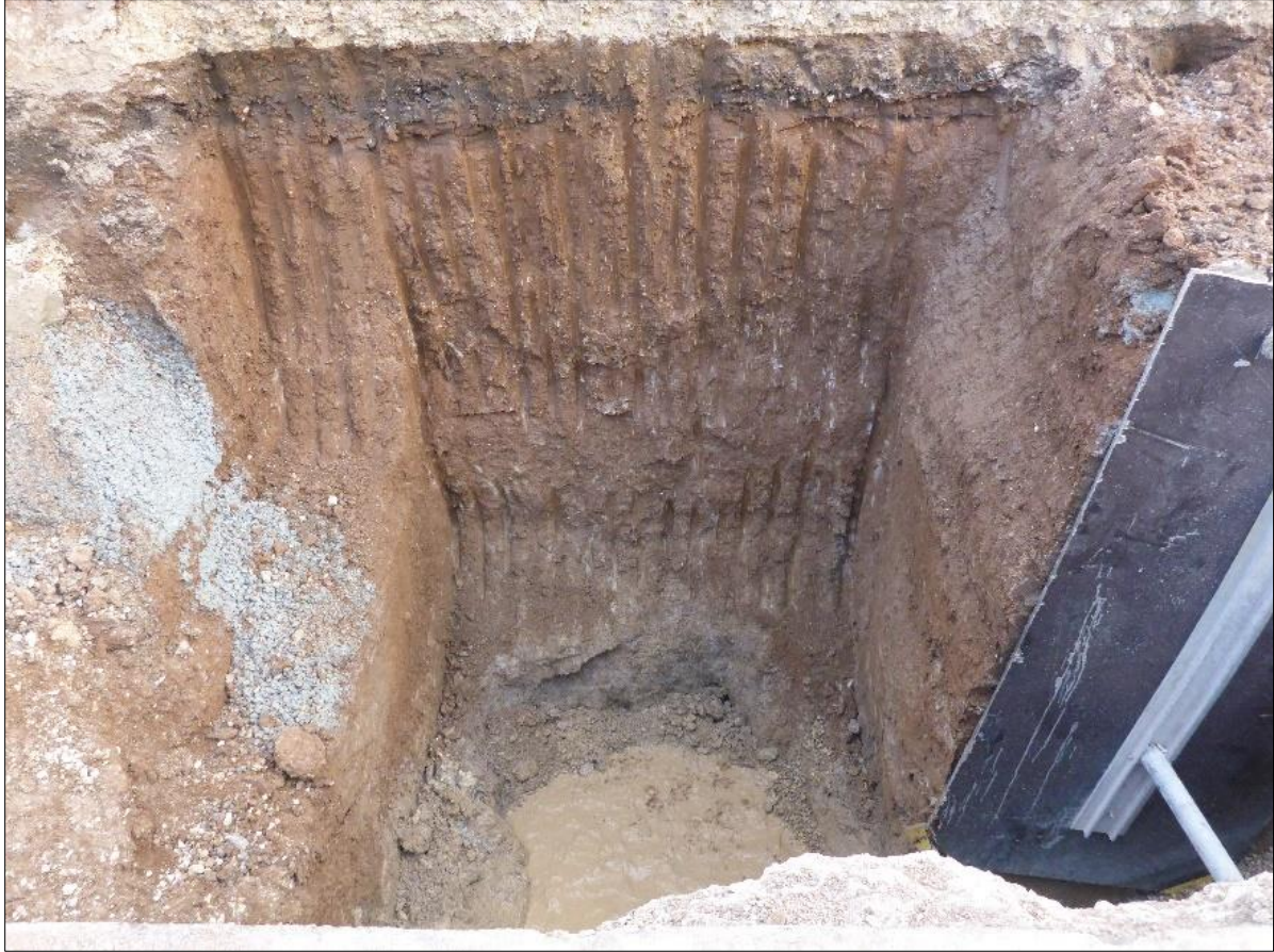
Figure 42. Trench profile of deepest, eastern portion of Exit Trench #2.
