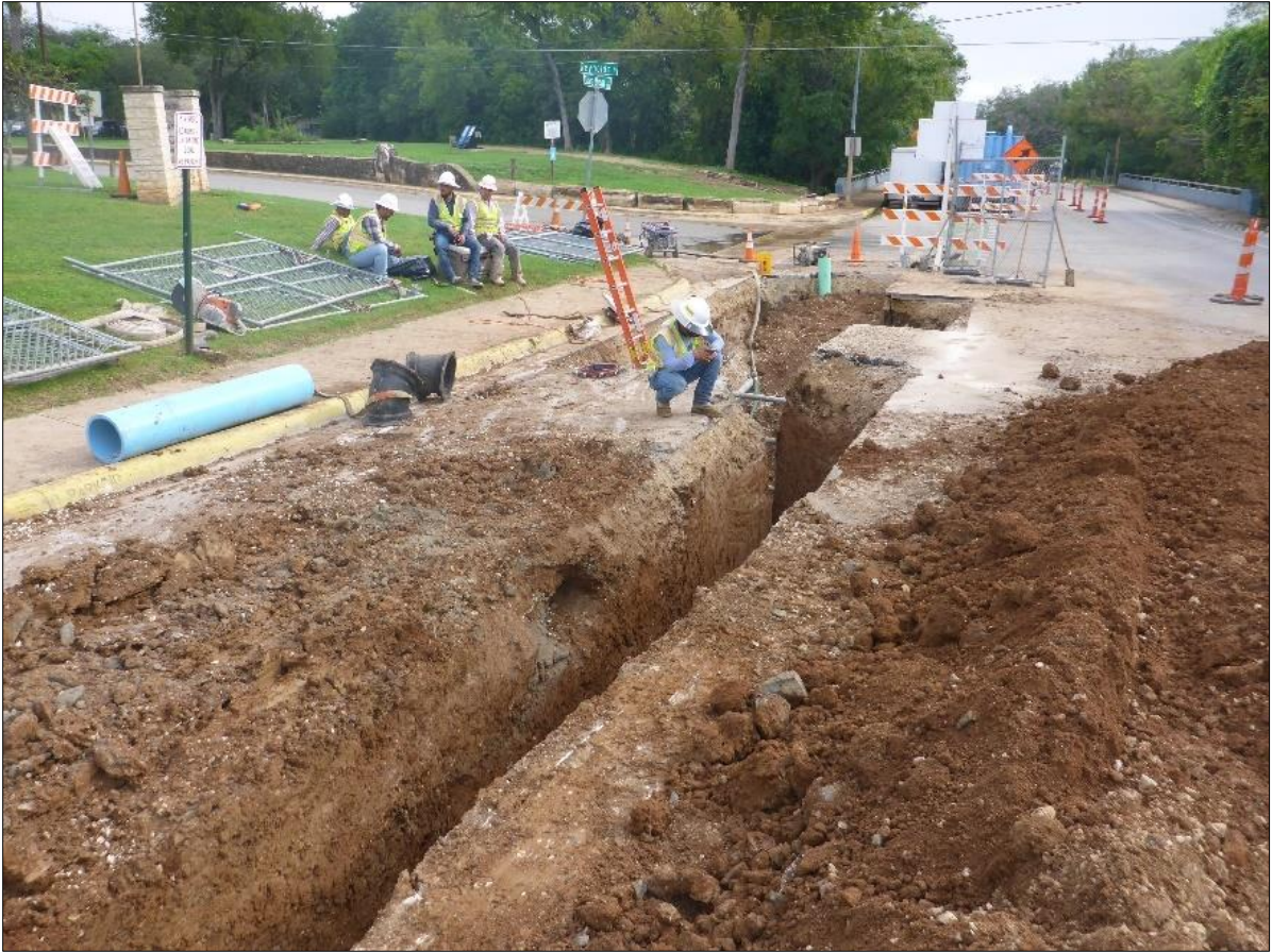
Figure 27. Exit Trench #2, on October 2 nd .
