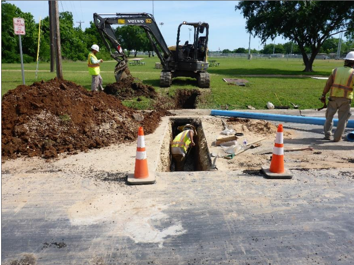
Figure 17. Waterline Offshoot Trench
