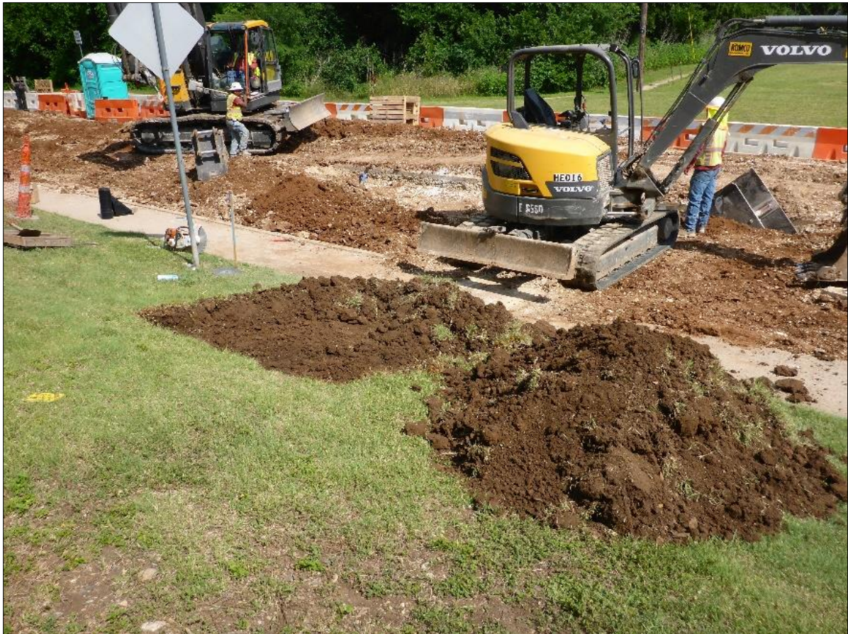
Figure 18. Manhole Access Box excavation on May 15 th .
