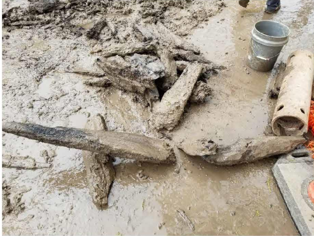
Figure 9. Wood from Trench.
