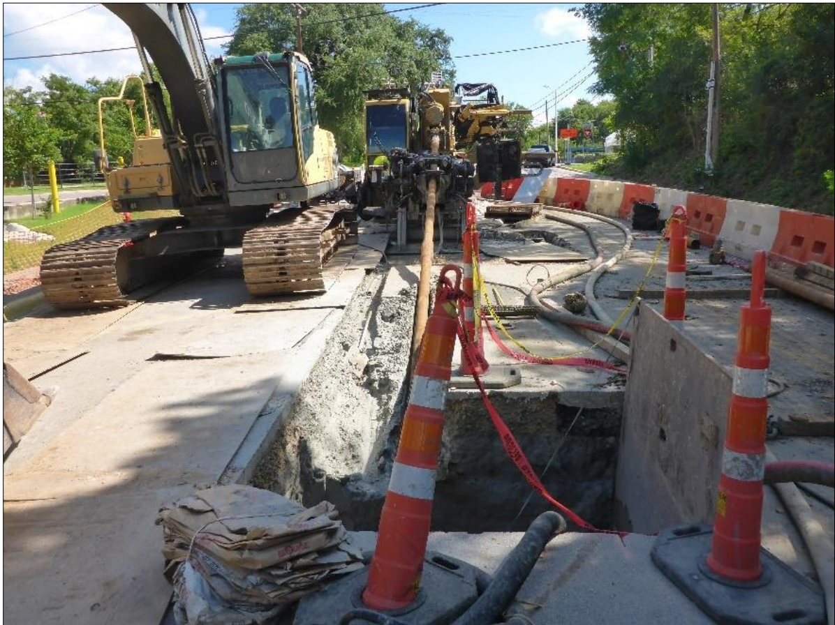
Figure 20. Entry Trench #2 with equipment staged around it, taken September 25 th .
