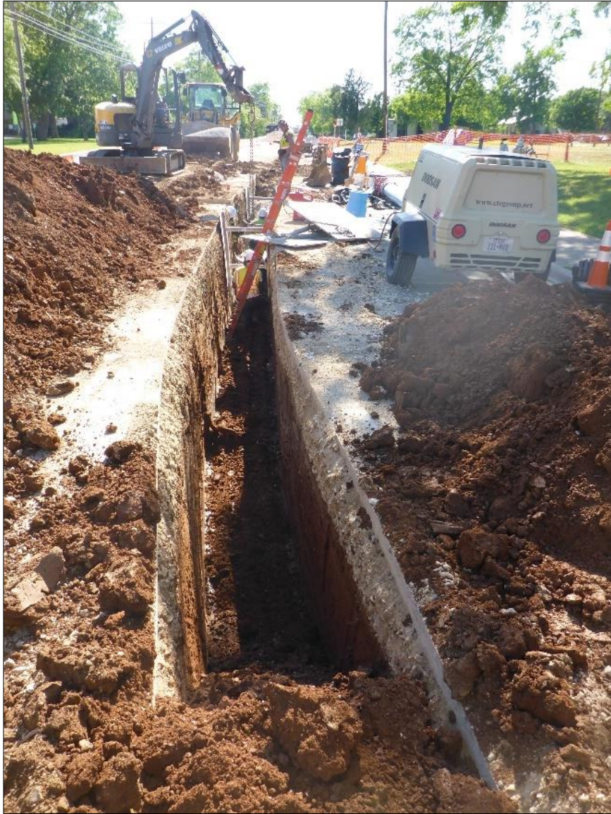
Figure 10. Waterline trench, taken on May 7 th .
