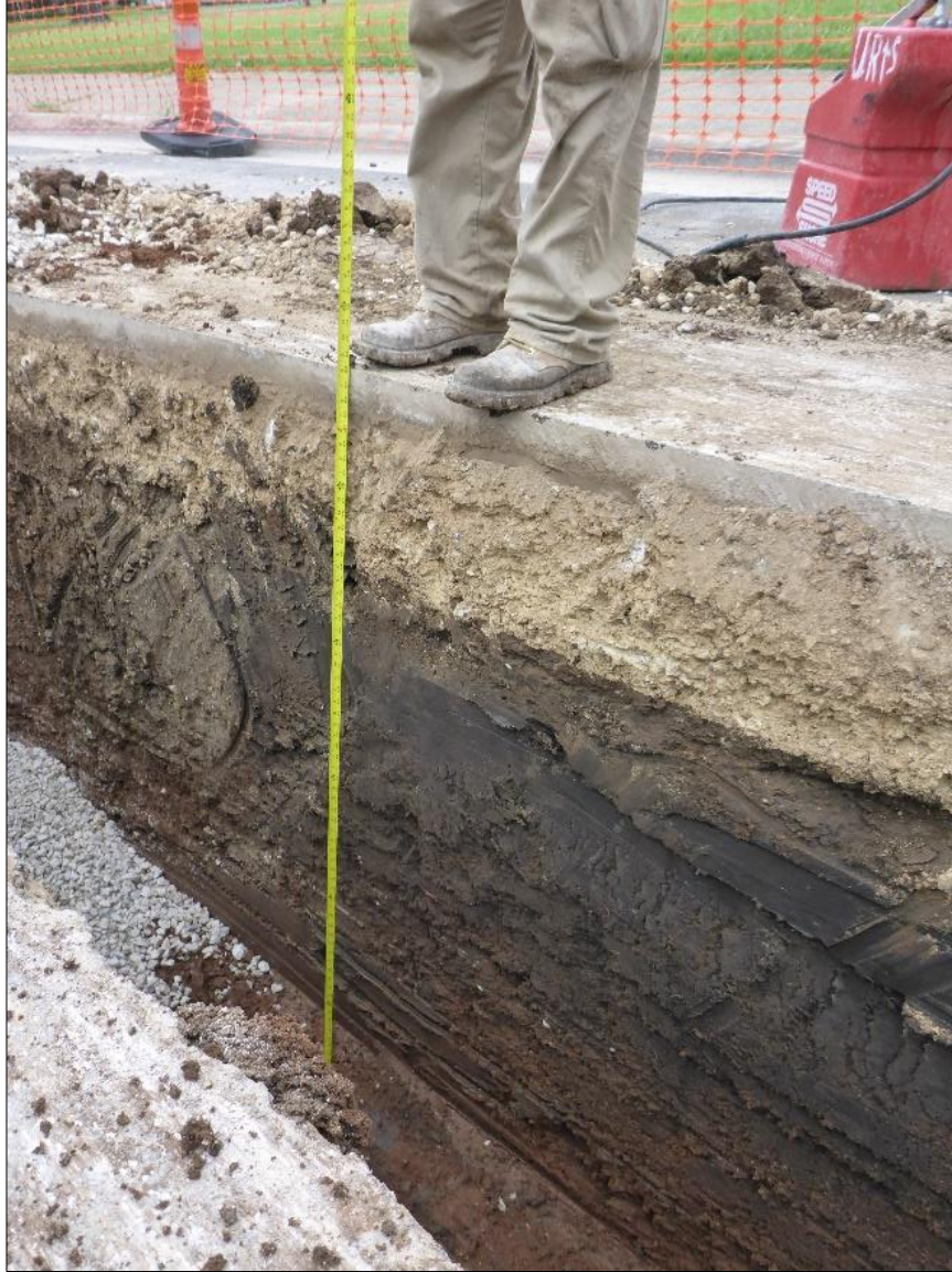
Figure 30. Waterline trench profile, taken on May 2 nd .
