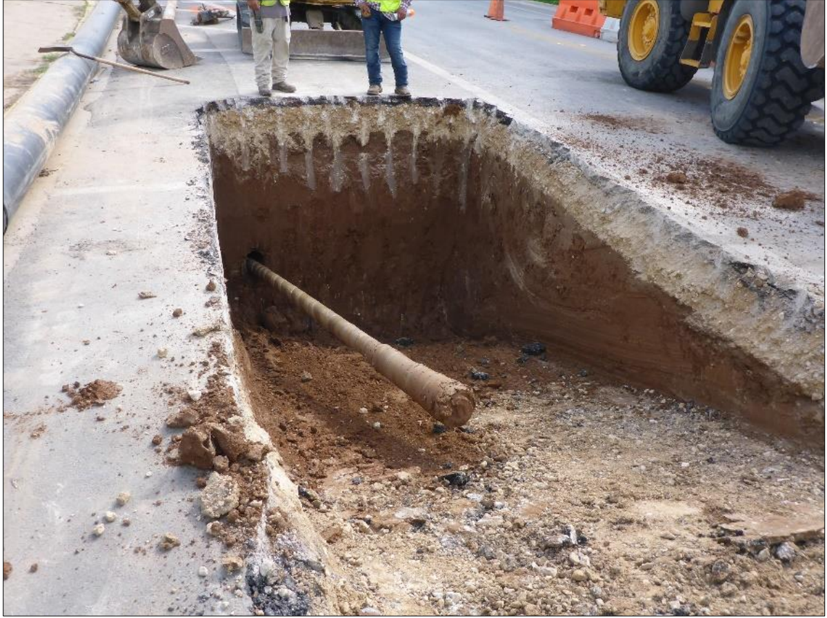
Figure 25. Exit Trench #2, on September 25 th .
