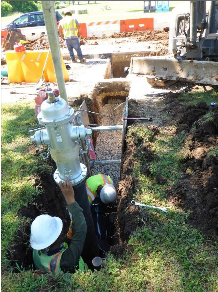
Figure 15. Fire Hydrant Trench, taken May 7 th .
