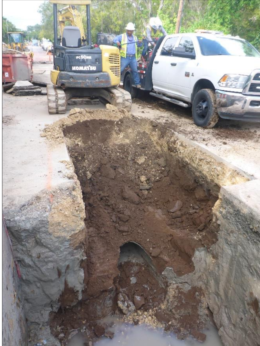
Figure 22. Expansion of Entry Trench #2 underway, on October 3 rd .
