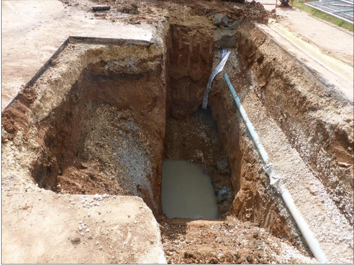
Figure 26. Exit Trench #2, on October 1 st .
