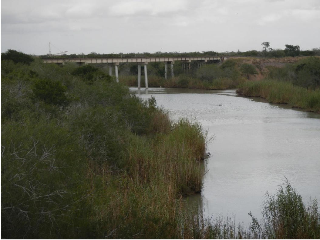
Figure 4. Arroyo Colorado overview, northeast
