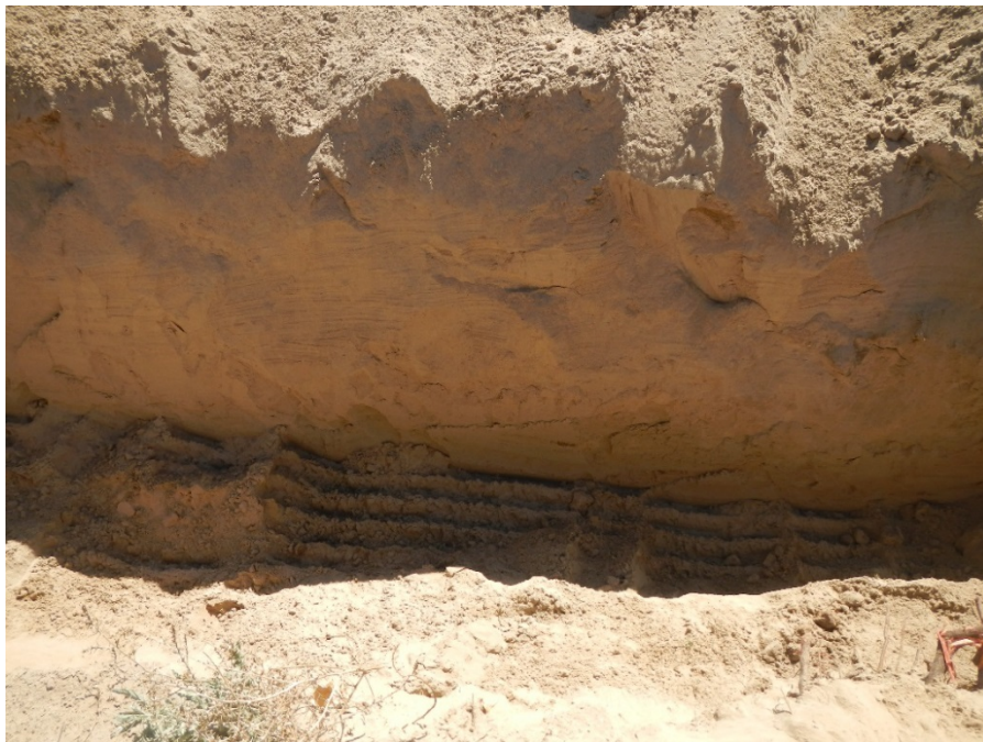
Figure 10. South wall of BHT 8.
