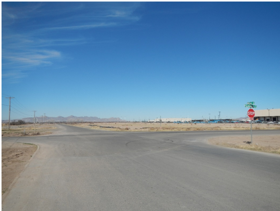
Figure 5. The existing Pan American Drive and Winn Road intersection; facing south.
