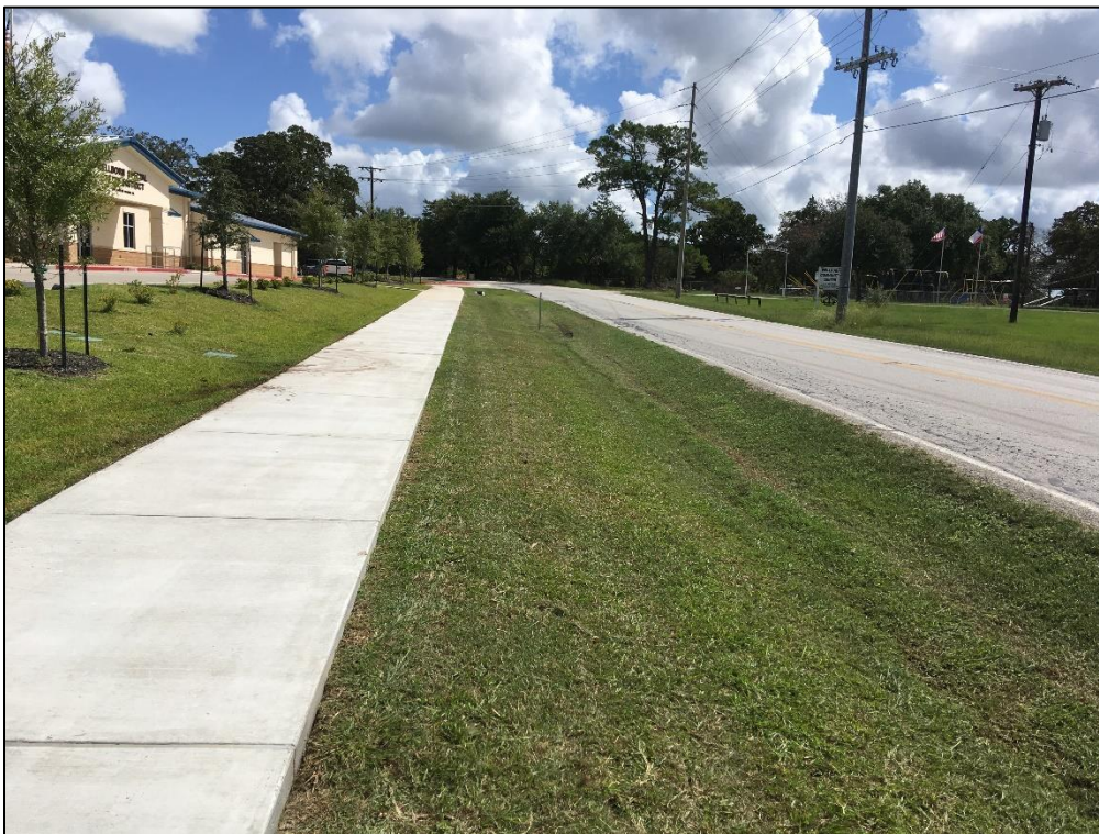
Photo 10. Southern portion of project area, western side of road. Note drainage ditch, maintained right-of-way, and sidewalk. View to the east.
