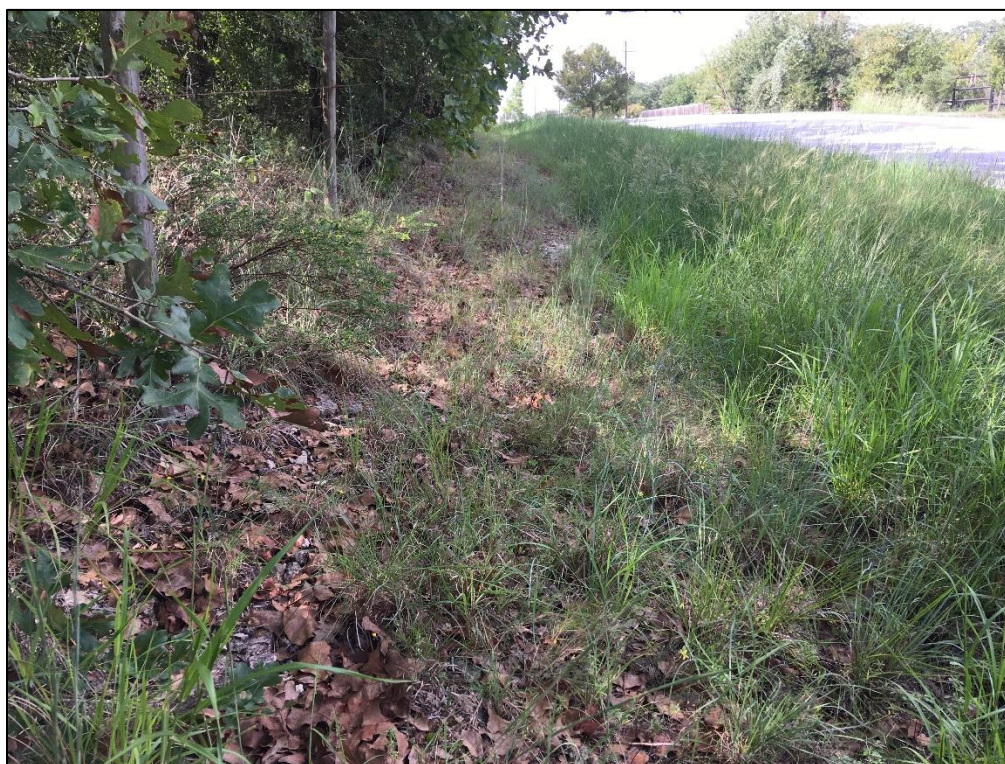
Photo 4. Northern portion of project area, eastern side of road. Note drainage ditch. View to the southwest.
