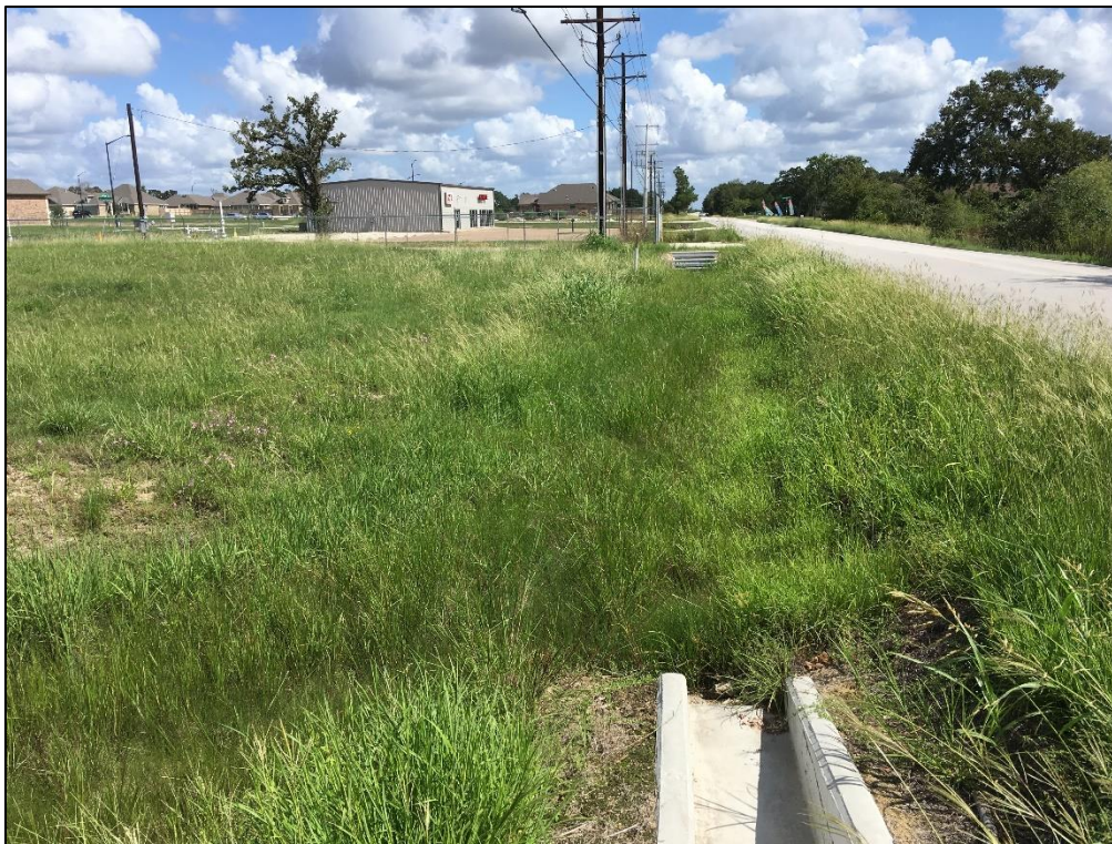
Photo 12. Central portion of project area, western side of road. Note drainage ditch. View to the northeast.
