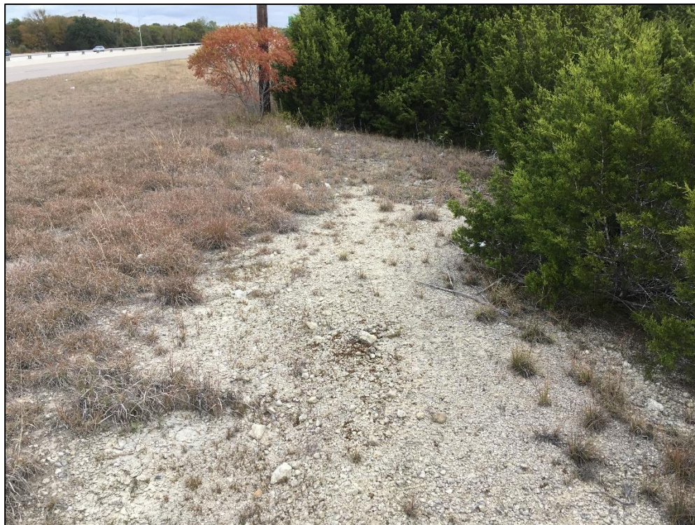
Photo 14. Central portion of project area. Note I-35 access road, caliche at surface. View to the northeast.
