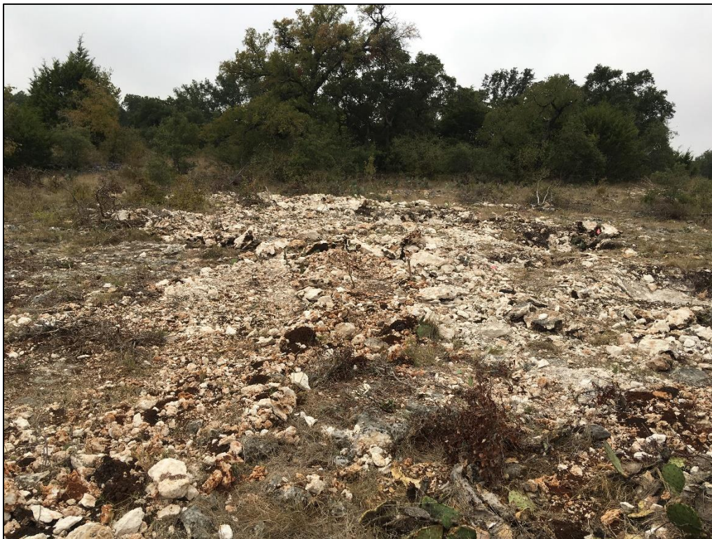
Photo 6. Backfilled excavated karst/sinkhole in the southwestern portion of the project area. View to the southeast.
