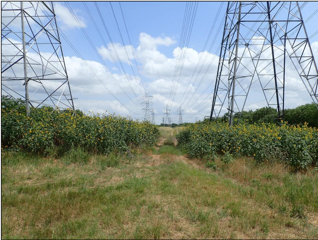
Figure 10 transmission line corridor within the project area, camera facing south
