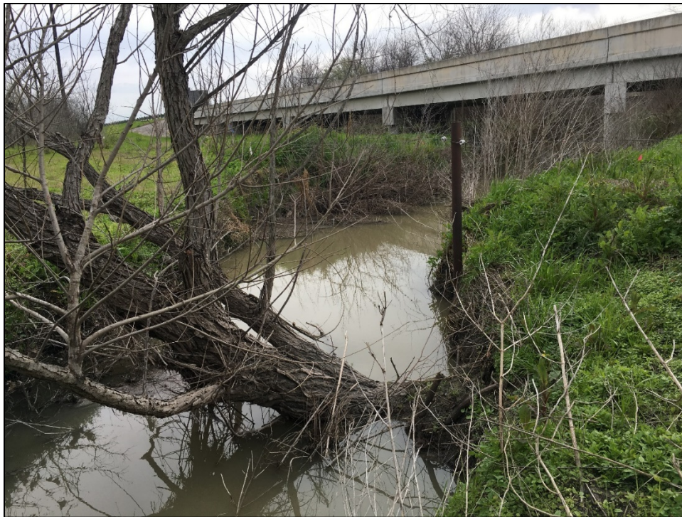
Figure 9. Photograph recorded on west bank of Salitrillo Creek facing IH-10 to the south, east of 41BX1693.
