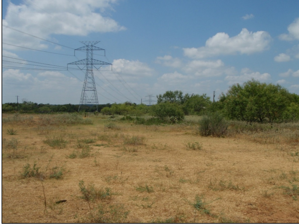
Figure 2. Overview of Site 41BP920, facing west.
