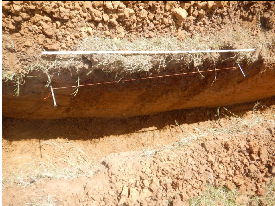
Figure 6. BHT01 overview and south wall profile, facing south.
