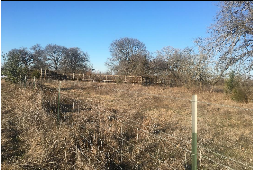
Figure 26. View of Resource 002, facing north
