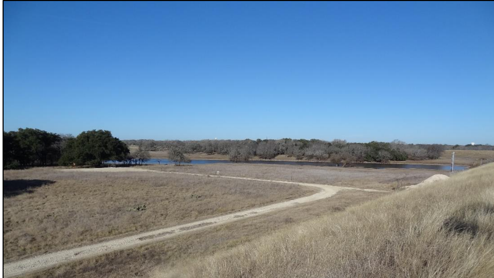
Figure 8. Overview of Dam No. 9 area, facing north
