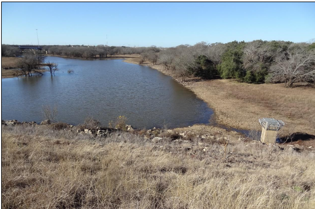
Figure 24. View from top of Dam No. 9, facing west
