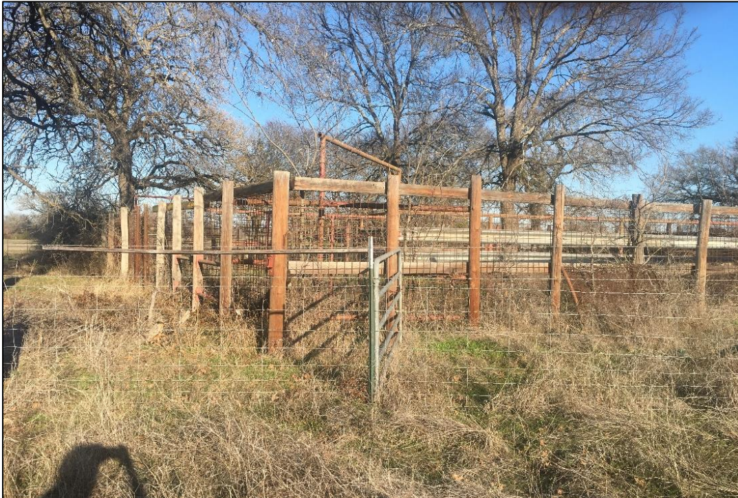
Figure 27. View of Resource 002 showing various construction materials, facing east
