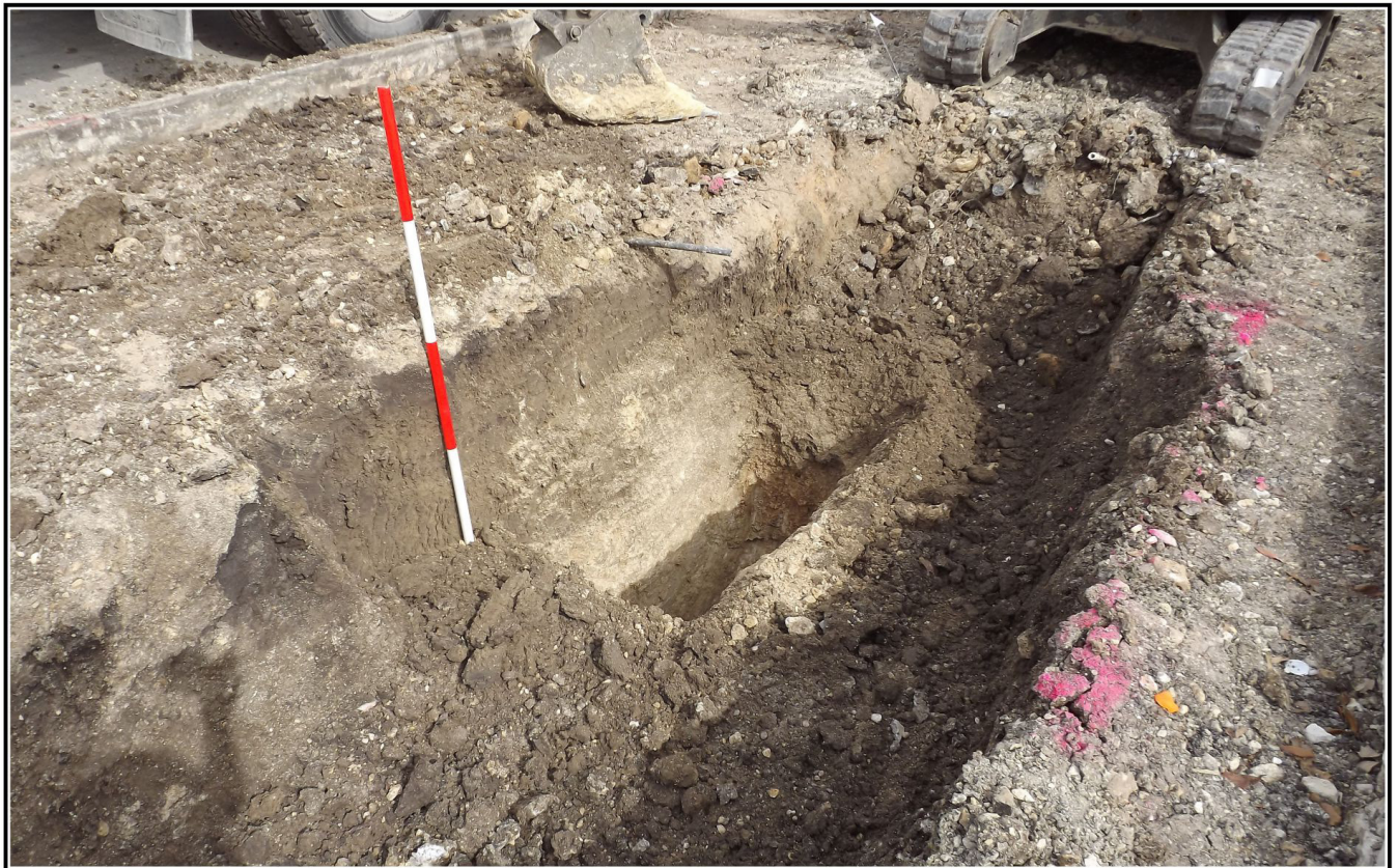
Figure 6-11. Typical pit excavation with deeper drainage pit against the wall and soil profile.
