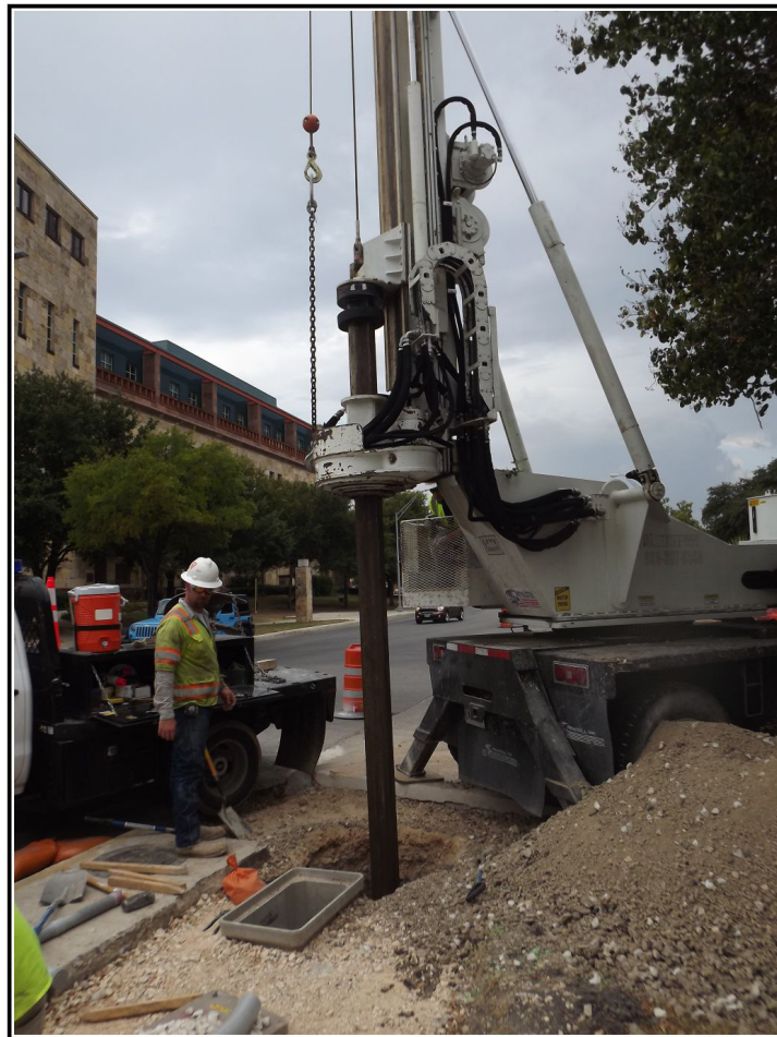
Figure 6-8. Excavation of the auger in Area 2 showing spoil pile.
