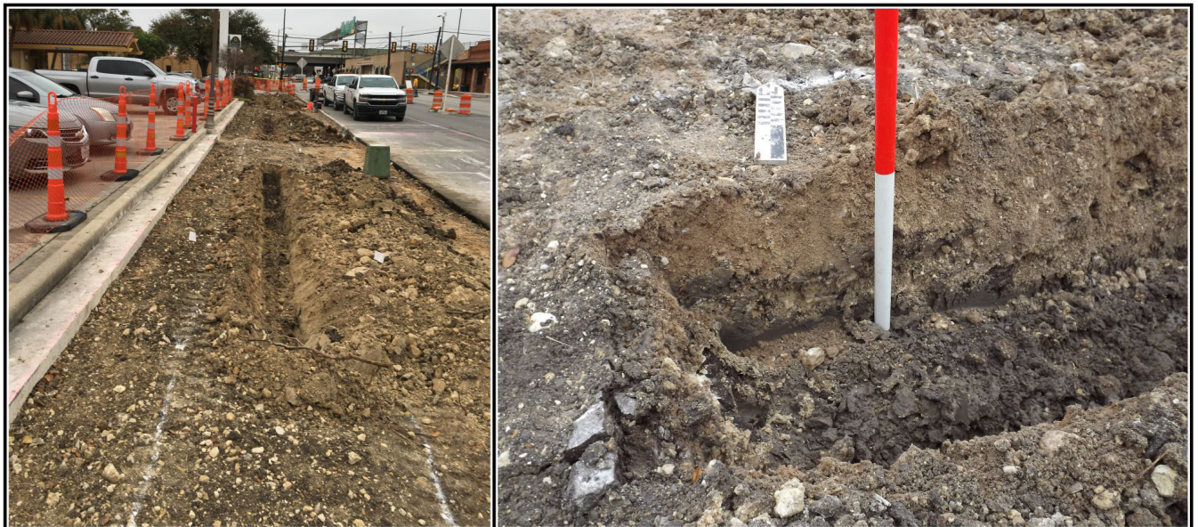
Figure 6-5. View to the west of the irrigation trench excavation with layout for planter boxes painted in white (left). Typical profile of irrigation wall view with construction fill to 25 cm (9.8 in.) below the grade followed by 5 cm (1.9 in.) of silty clay (right).
