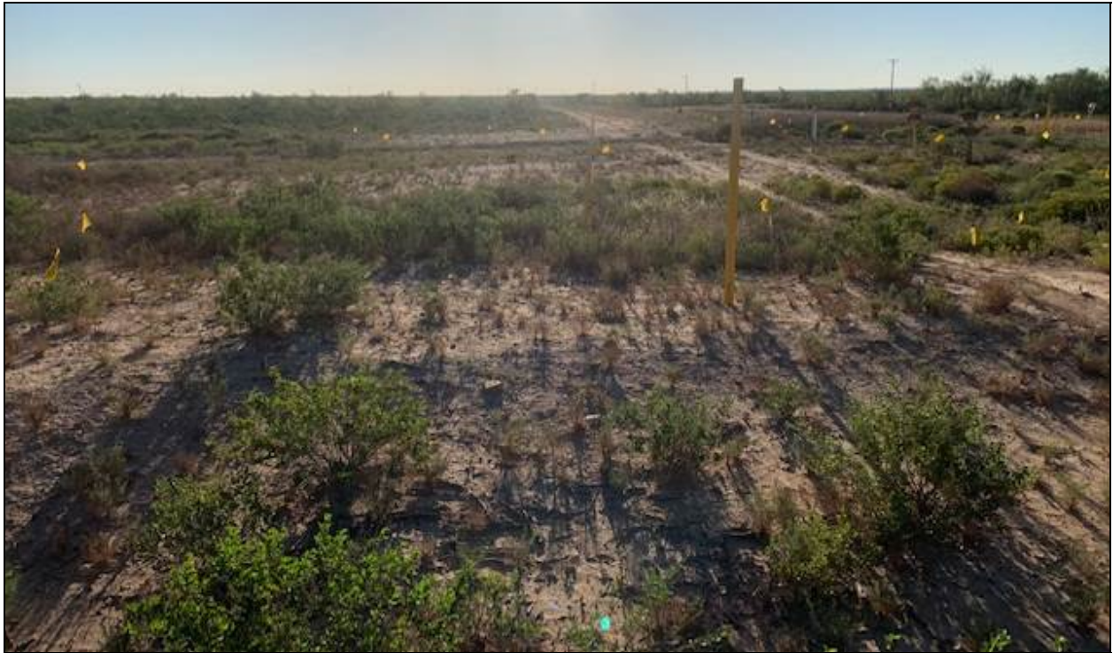
Figure 6-1. Existing pipeline parallel to the current Project Area (facing southeast)
