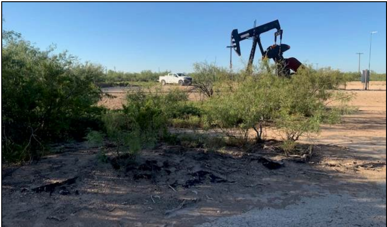
Figure 6-4. Existing pumpjack and pad in central portion of Project Area (facing south)
