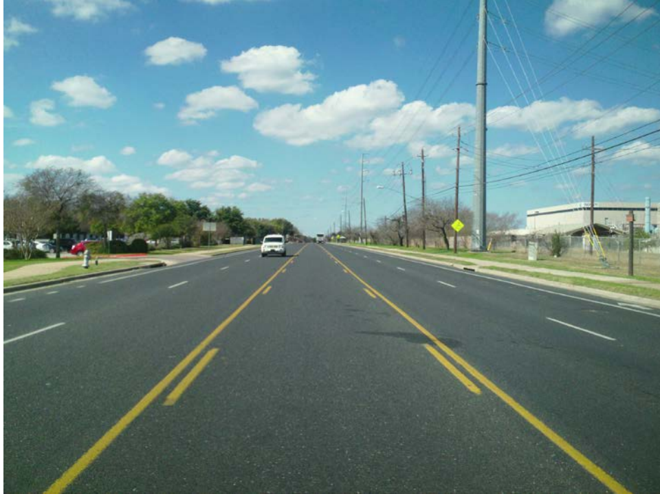
Figure 8: Urban setting of proposed alignment along East Oltorf Street, facing west.
