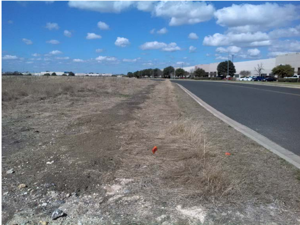
Figure 12: Overview of southern terminus of proposed alignment at Trade Center Drive looking north.
