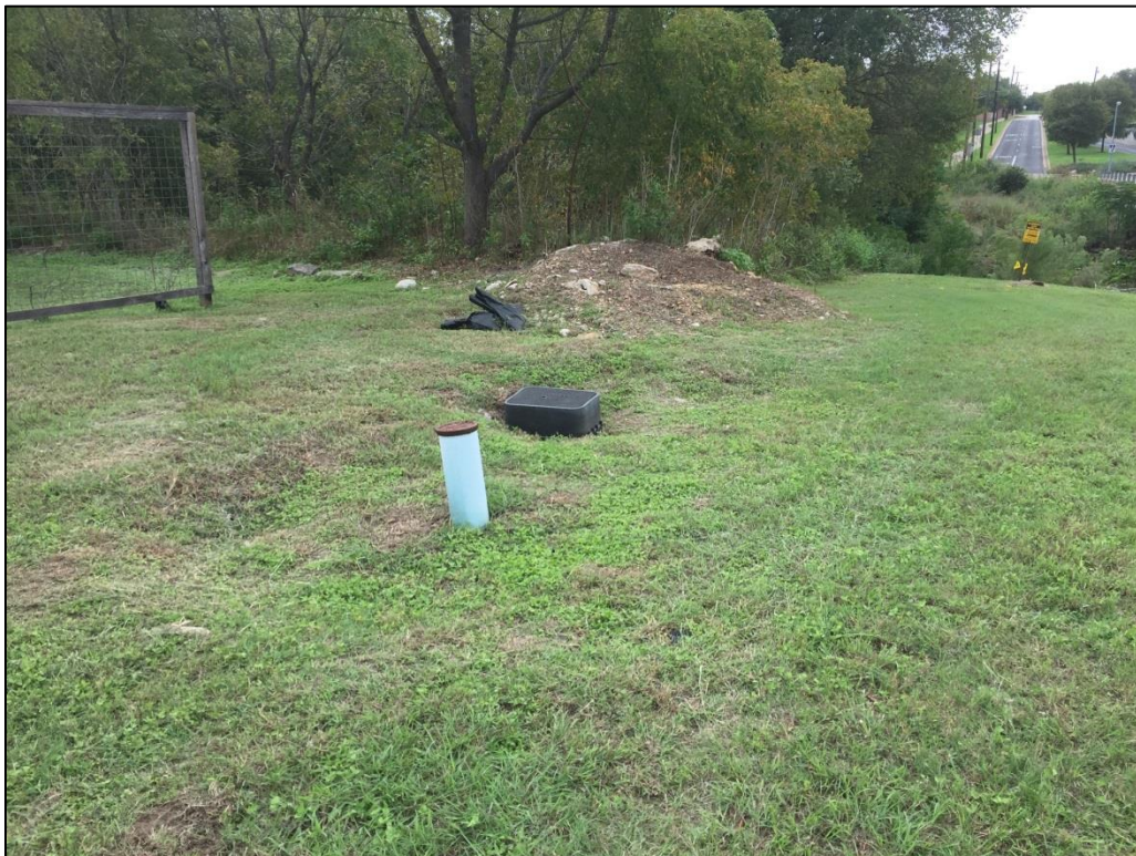
Figure 17. Buried water lines in ROW on east side of Great Oaks Drive Bridge.
