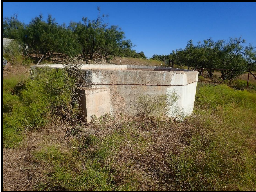
Figure 12. Octagonal concrete water cistern at site 41SC76, facing north
