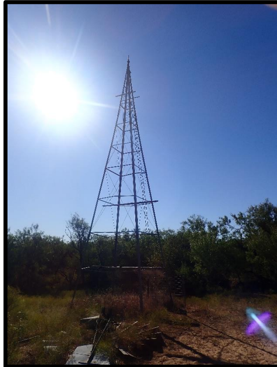
Figure 11. Site 41SC76 windmill structure and motor in the foreground, facing south
