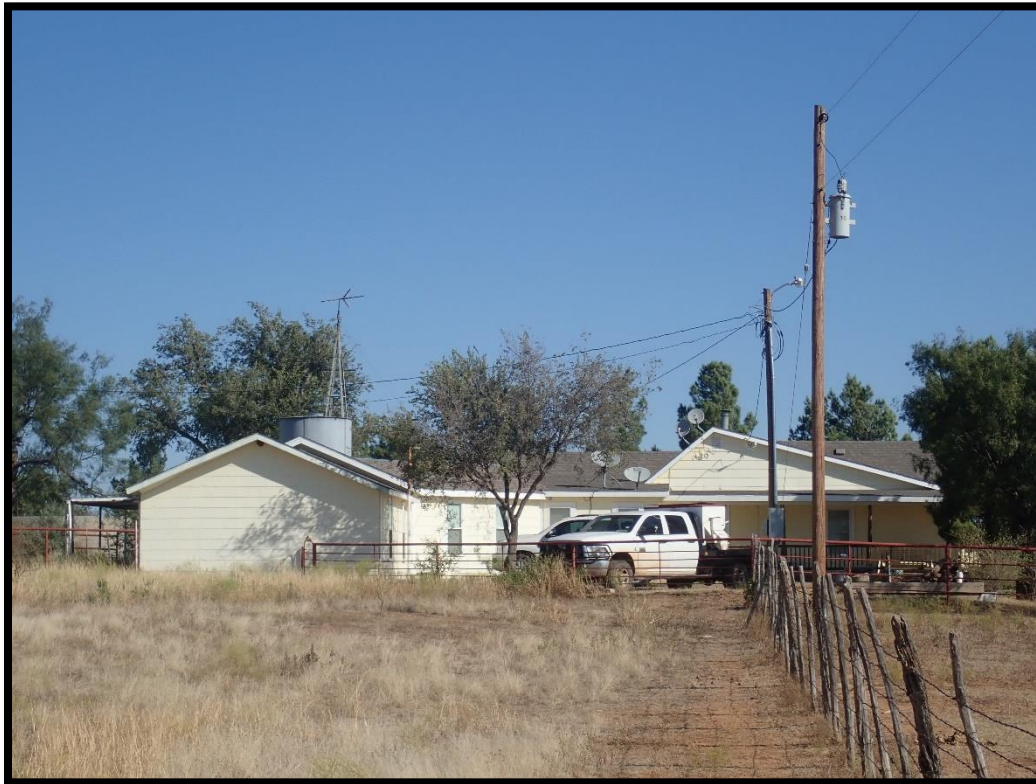
Figure 25. View of Resource 001a, facing north
