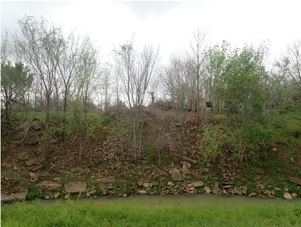
Figure 5-4. Residential property and riprap along Buffalo Bayou, view is facing southwest.
