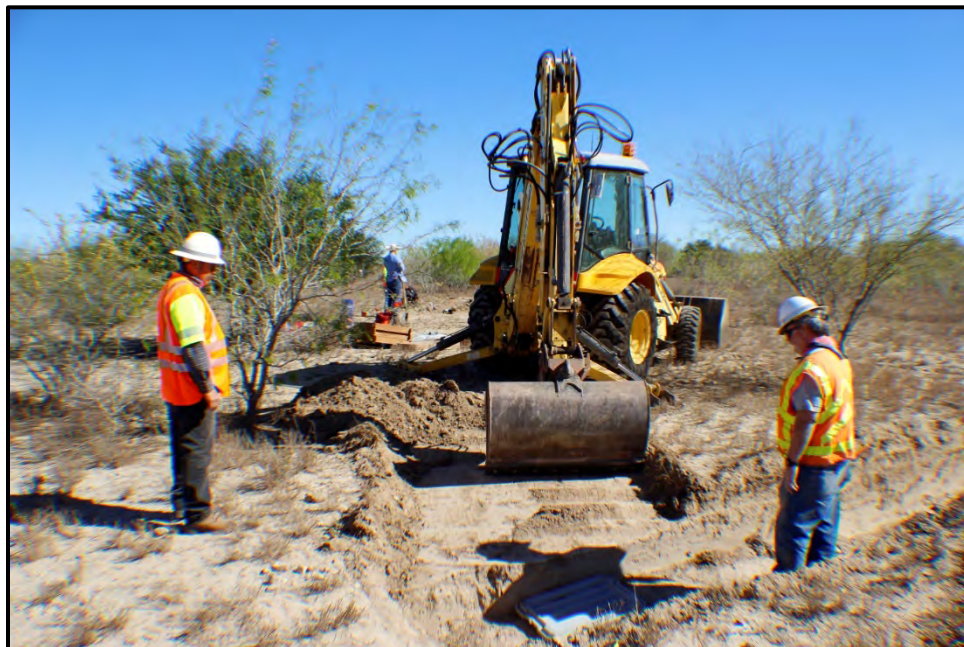
Figure 5.2. Crew removing overburden during backhoe trench testing, facing east.
