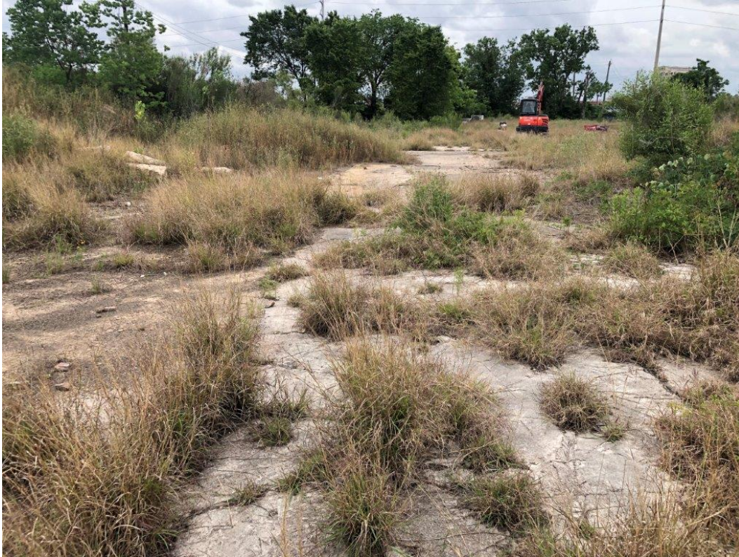
FIGURE 9: VIEW OF MODERN FOUNDATION REMNANTS, FACING SOUTH
