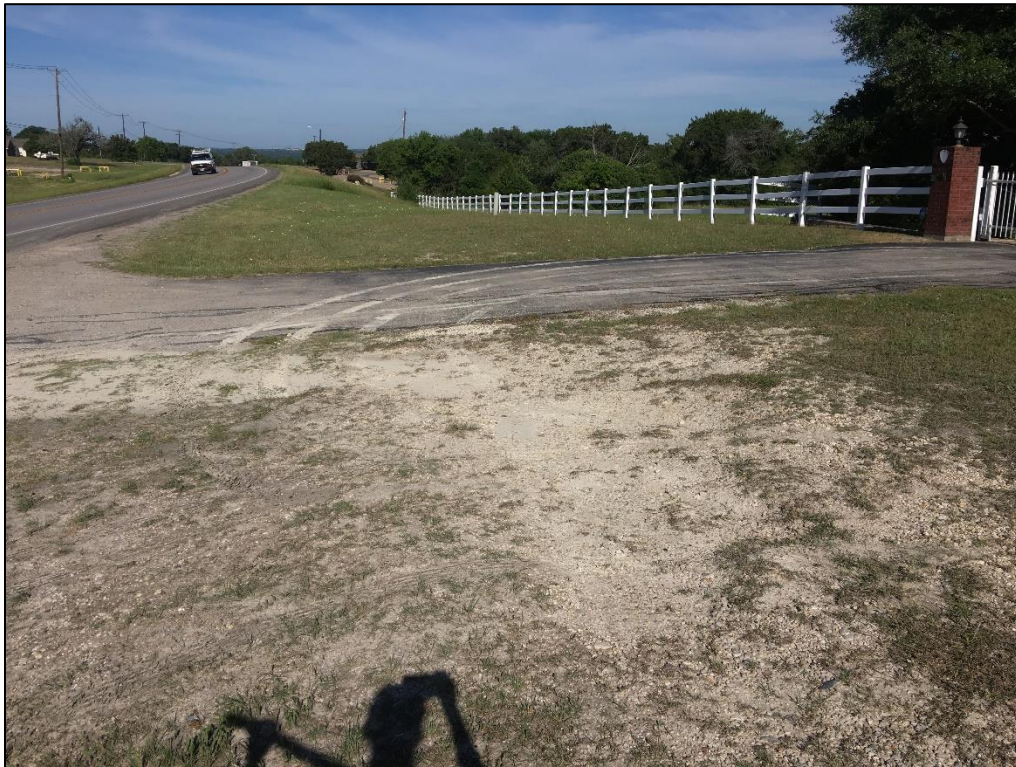
Photo 21. Northern side of FM 93, western end of alignment. Note gravels at surface. View to the west.
