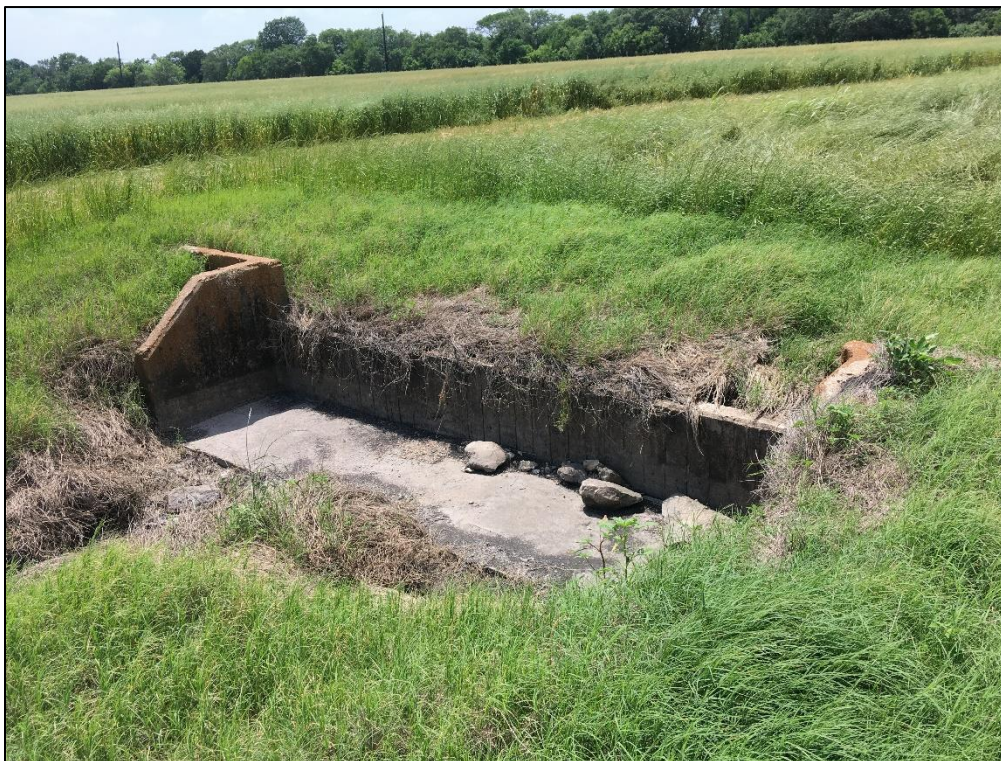
Photo 30. Isolated Find 05. Concrete spillway in channelized drainage. View to the southwest.
