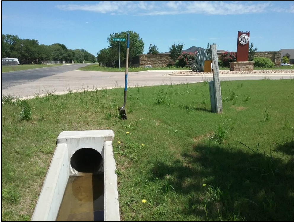
Photo 15. Eastern side of Hartrick Bluff Road, north of ML28. Note drainages, roadway, buried utility marker near wooded pole. View to the north.
