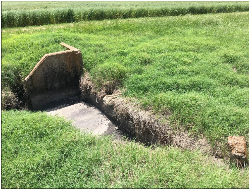
Photo 29. Isolated Find 04. Concrete spillway in channelized drainage. View to the southwest.
