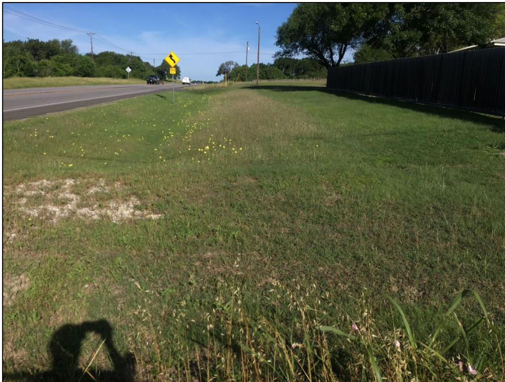
Photo 20. Northern side of FM 93, west of CG37. Note drainage ditch. View to the west.
