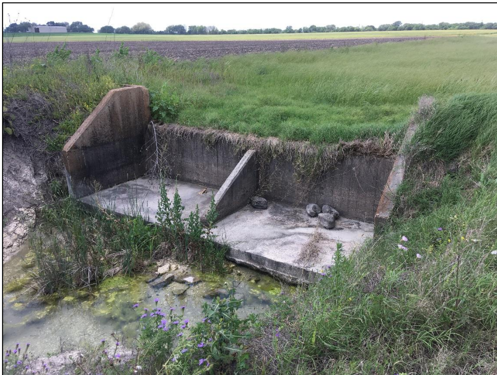
Photo 28. Isolated Find 03. Concrete spillway in channelized drainage. View to the southwest.
