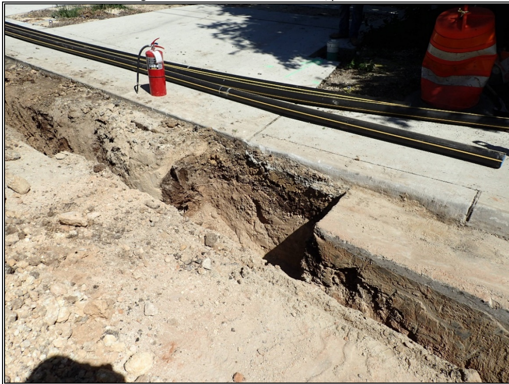
Figure 26. Southern terminus of LSET 6 at tie-in to ML 1, facing northwest.
