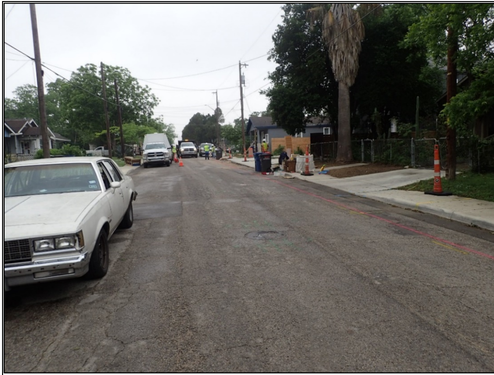
Figure 4. Overview of the Project Area near the eastern terminus, facing west.
