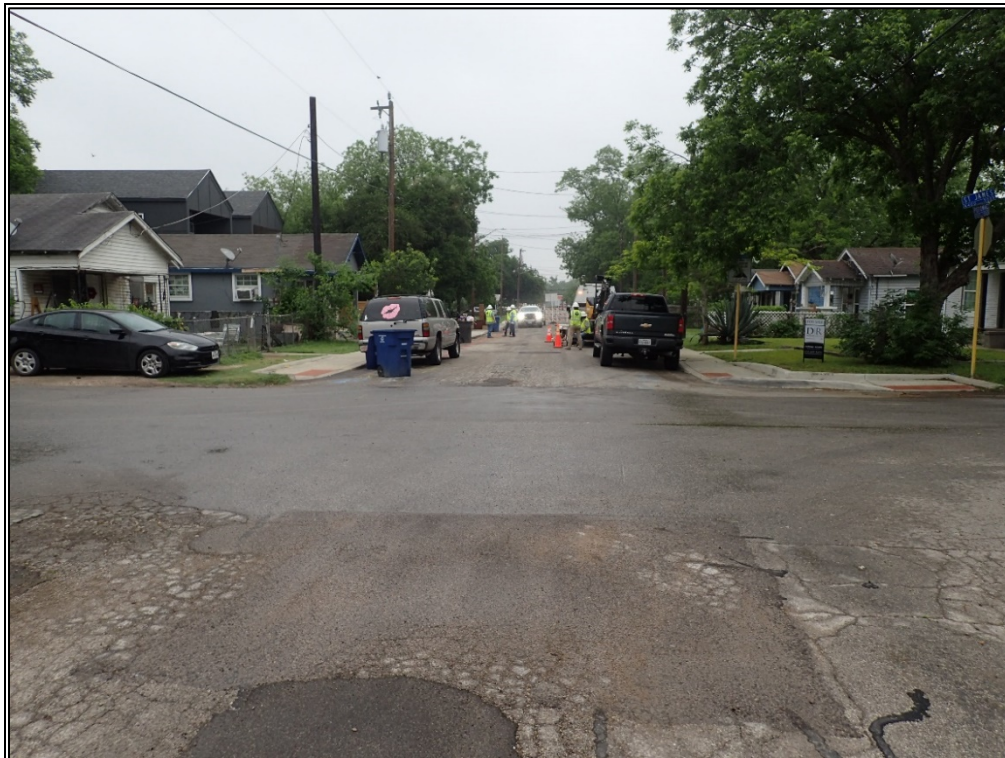
Figure 3. Overview of the Project Area near the western terminus at the St. James Road and Potomac Street intersection, facing east.
