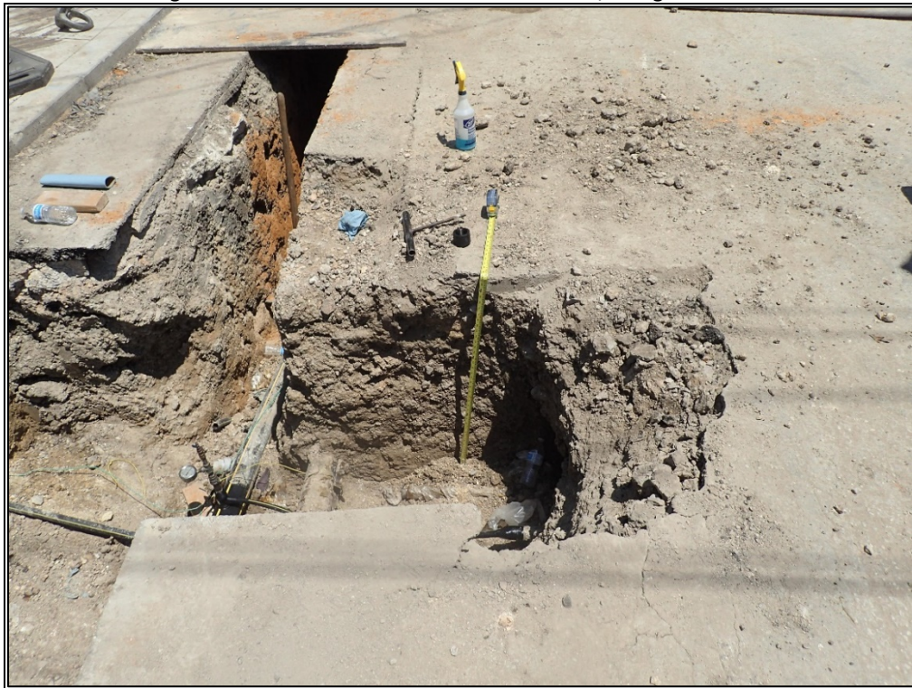
Figure 22. North portion of LSET 3 at tie-in with ML 1, facing east.
