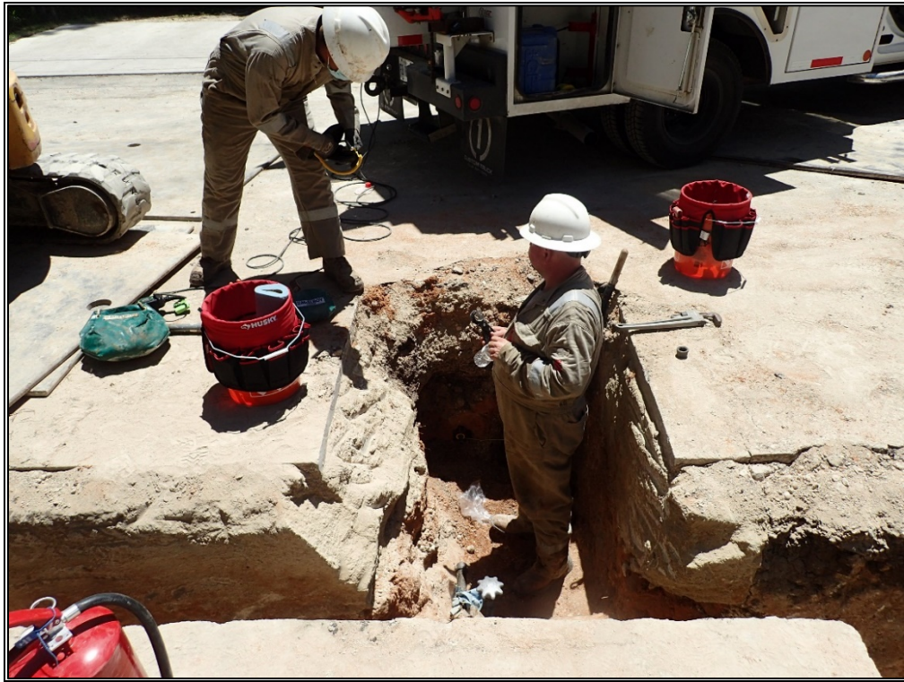
Figure 23. LSET 4 at old ML connection, facing south.
