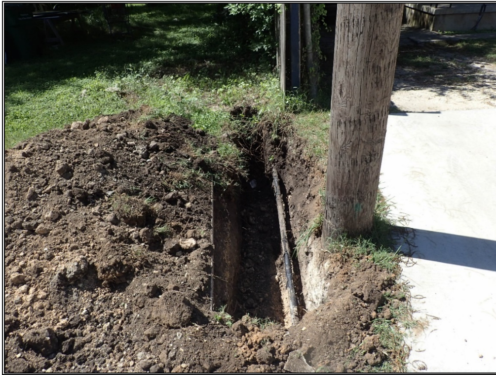
Figure 29. LSET 7 on south side of Potomac Street, facing south.
