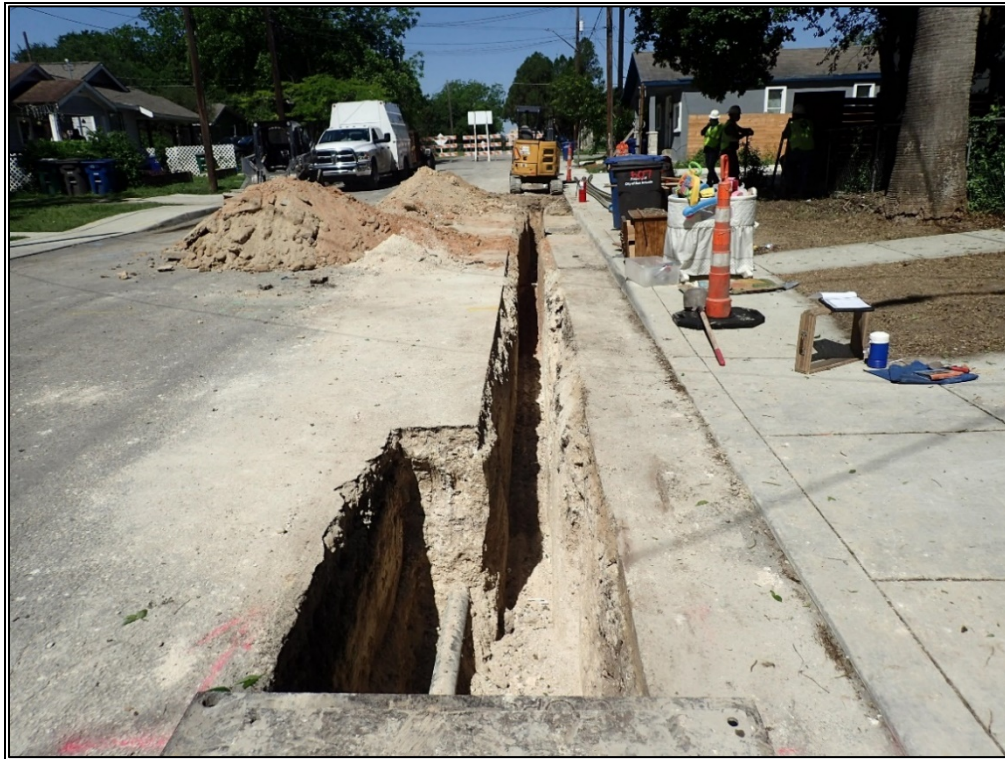
Figure 17. Overview of ML 1 trench from eastern terminus, facing west.
