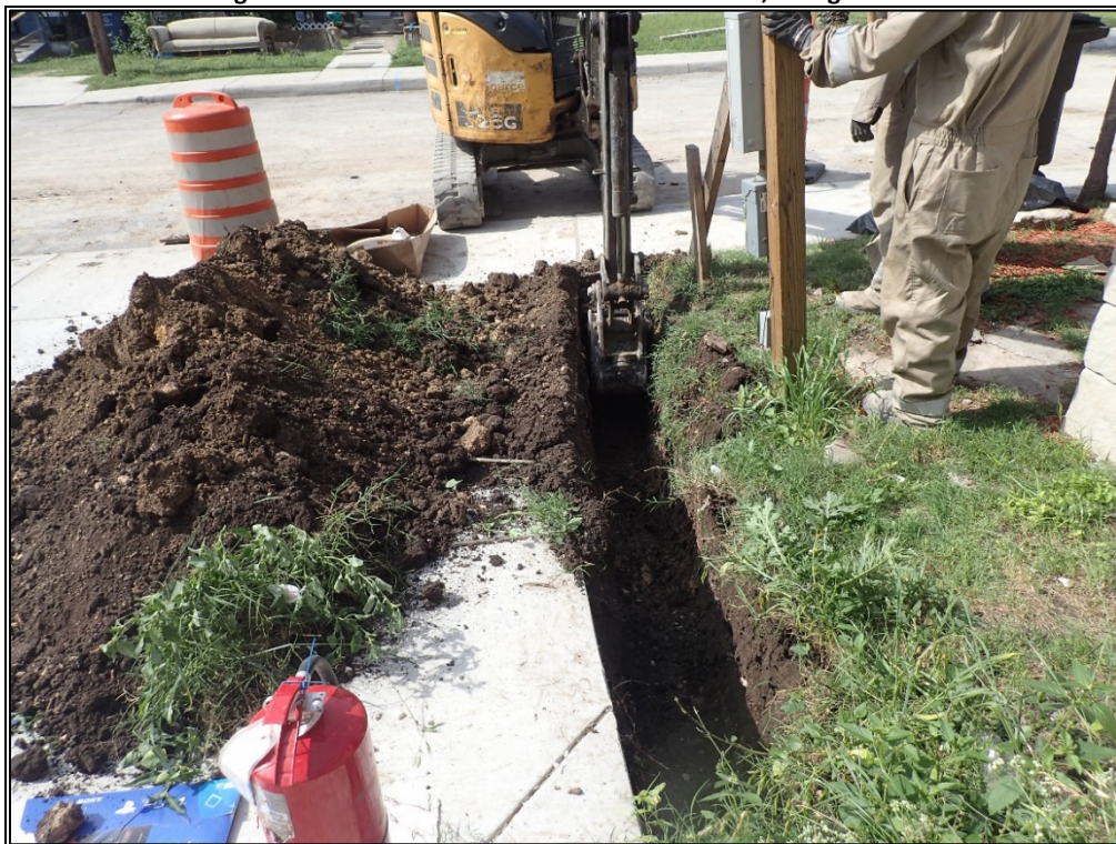
Figure 30. Overview of LSET 8, facing south.
