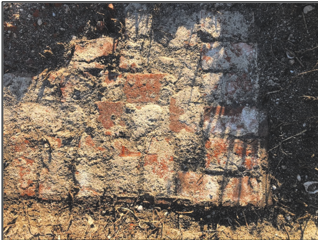
Figure 5.35b. Detail of brick chimney base, Northeast corner.
