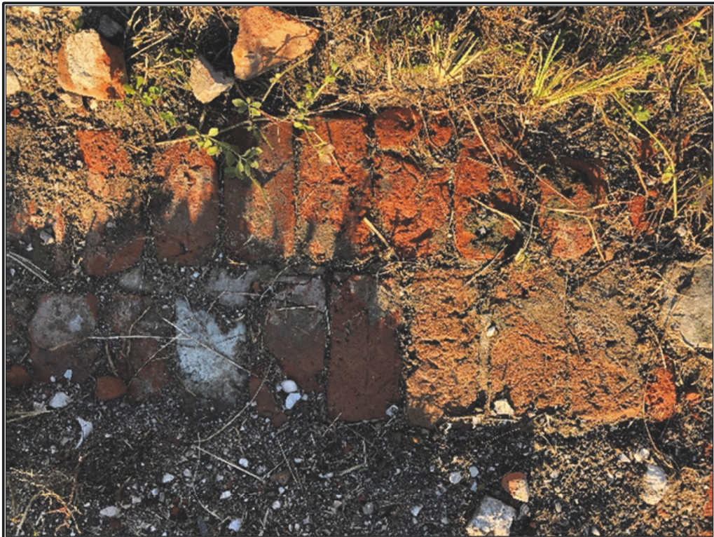
Figure 5.32b. East wall at Southeast corner of foundation, looking west.
