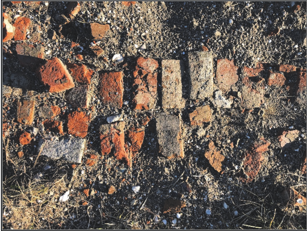
Figure 5.30a. Detail of North wall at Northeast corner of foundation, looking south.
