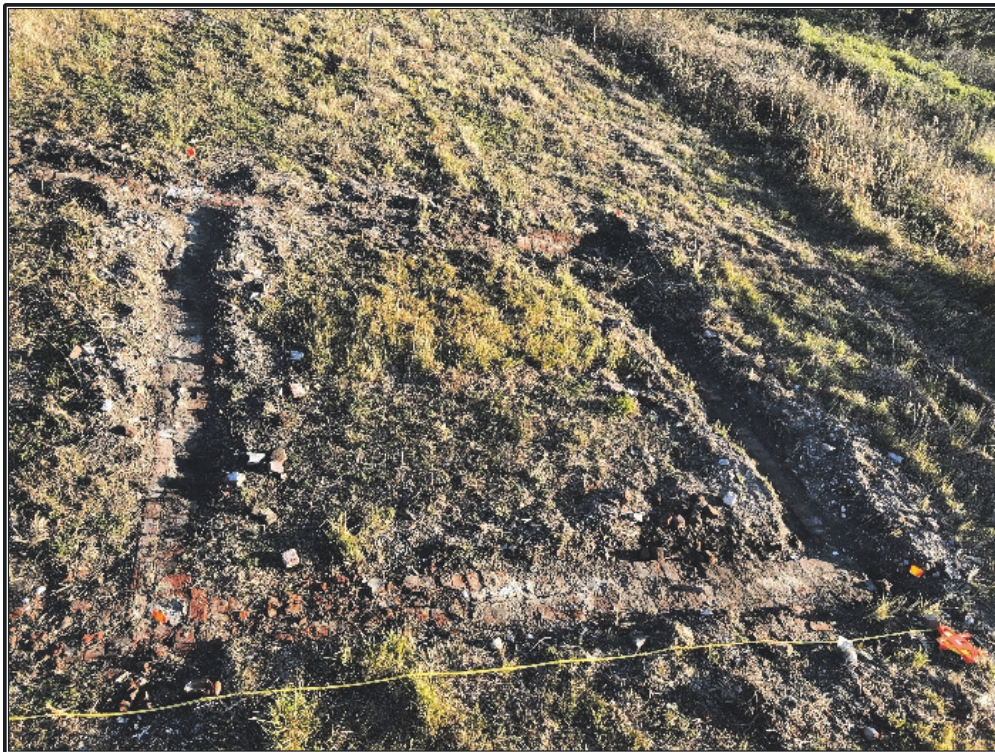
Figure 5.28b. Photo of exposed rectangular brick foundation (from atop ladder) –West side - looking south; cross wall is shown in photo.
