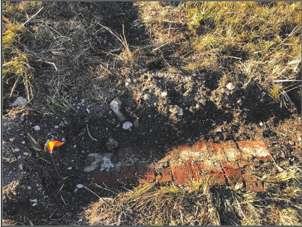
Figure 5.31a. Southwest corner of foundation, looking north.
