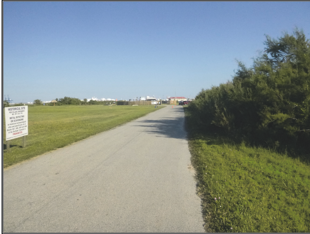
Figure 2.1. Overview of the eastern portion of the survey area, view to the northwest from the survey grid origin at the eastern corner of the project area.
