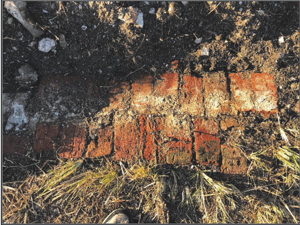
Figure 5.32a. Detail of South wall at Southwest corner of foundation, looking north.
