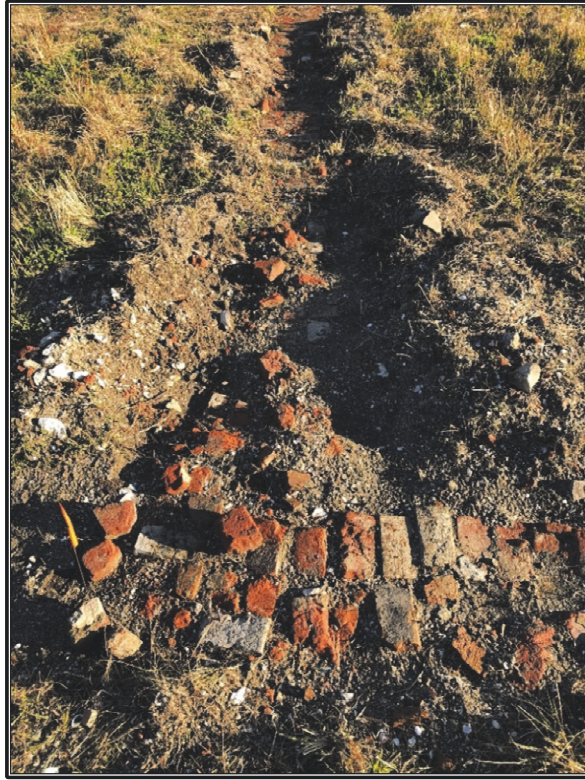
Figure 5.29a. Northeast corner of foundation, looking south.
