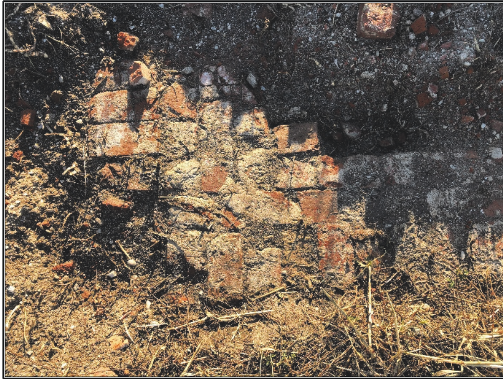
Figure 5.35a. Detail of brick chimney base, Southeast corner.
