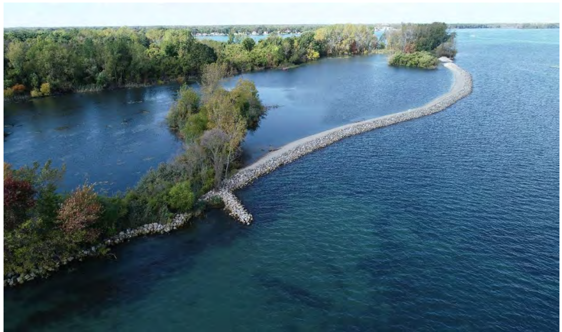
Figure 3. A new habitat shoal protects fragile coastal wetlands at Celeron Island's north bay from further erosion and enhances this backwater area for fish spawning and nursery activity (credit: Friends of the Detroit River).
