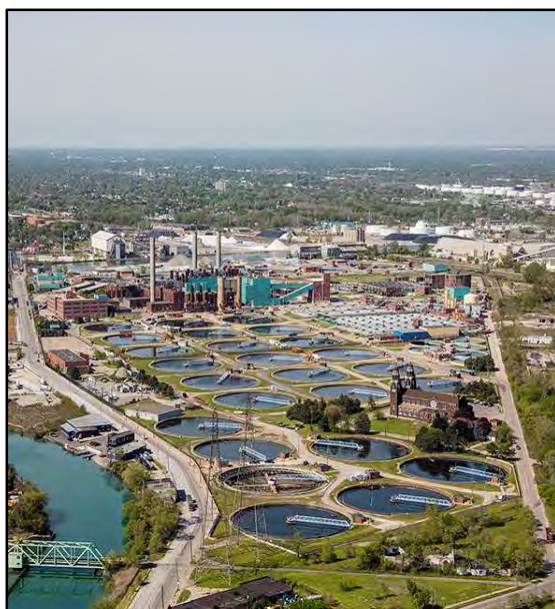
Figure 1. An aerial photograph of GLWA's Water Resource Recovery Facility - one of the largest in North America (credit: GLWA).
